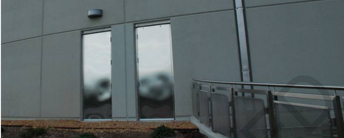
Figure 3-4 Emergency Exit Doors
