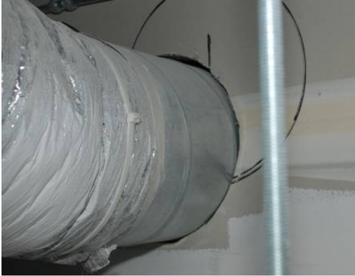
Figure 3-6 Sealing Penetrations
