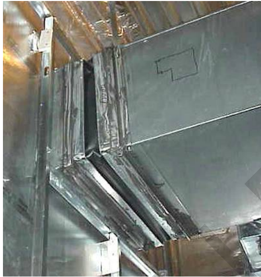
Figure 3-5 Duct Penetrations
