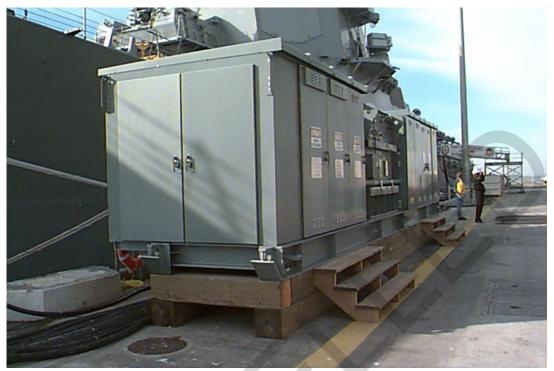
Picture C. A skid-mounted substation
