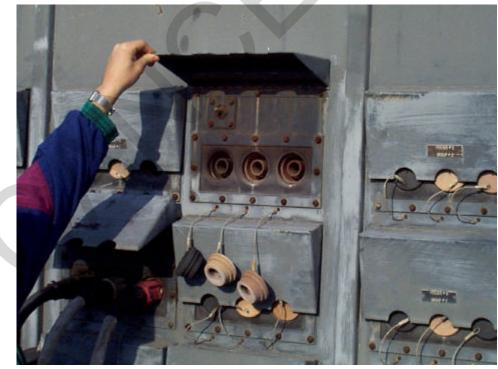
Picture D. A skid-mounted substation with camlock connections.
