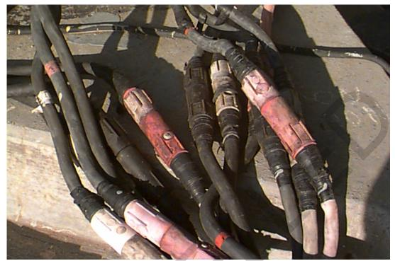
Picture I. A 480-volt shore-cable to ship-cable with camlock connection.
