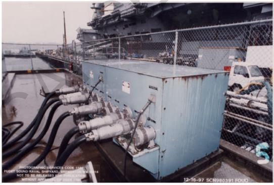
Picture F. A 4.16-kV pier electrical outlet assembly and outlets.
