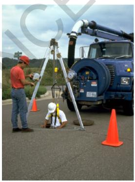
Picture M. **Effective vault rescue.** (Courtesy of DBI/Sala)
