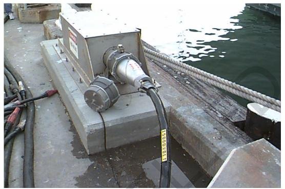
Picture A. Electrical connection outlet assembly with a 15-kV receptacle.
