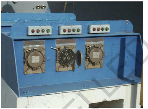
Picture E. A 480-volt pier electrical outlet assembly without cable connections.
