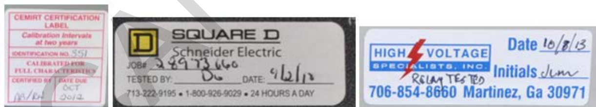
Figure 1-5 Typical Calibration or Maintenance Stickers
