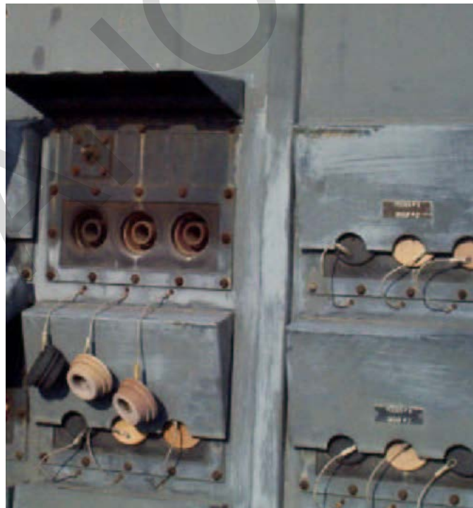
Figure 12-5. Skid-Mounted Substation with Single-Pole Connections
