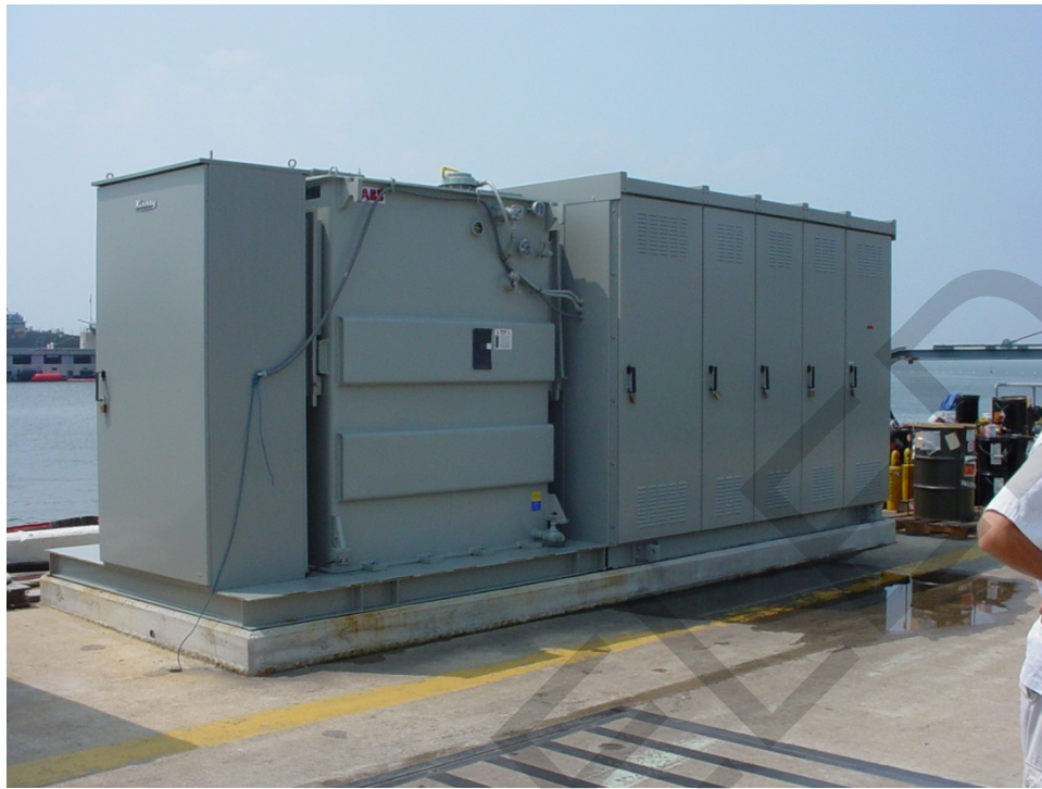
Figure 12-5. Skid-Mounted Substation with Single-Pole Connections
