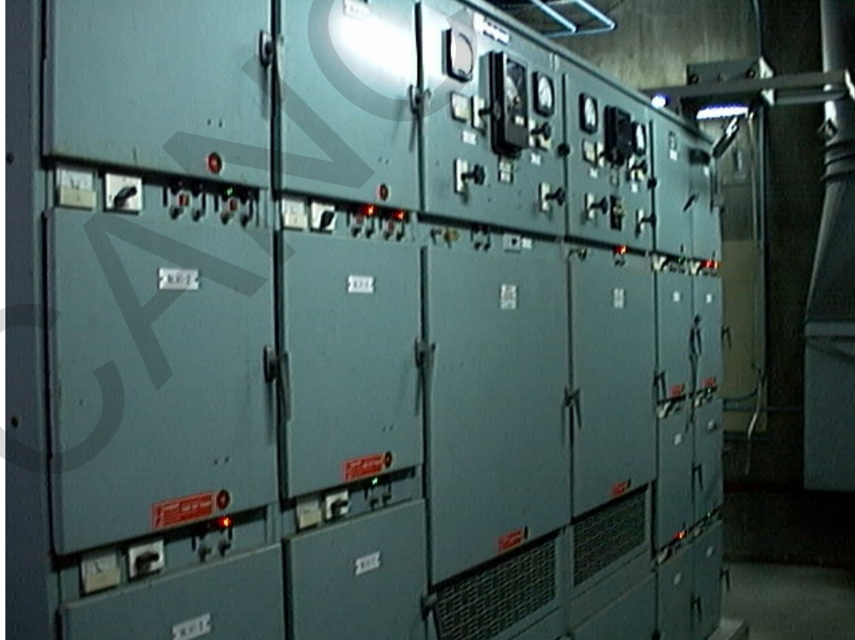
Figure 12-3. Inside a Pier Vault Housing a Substation
