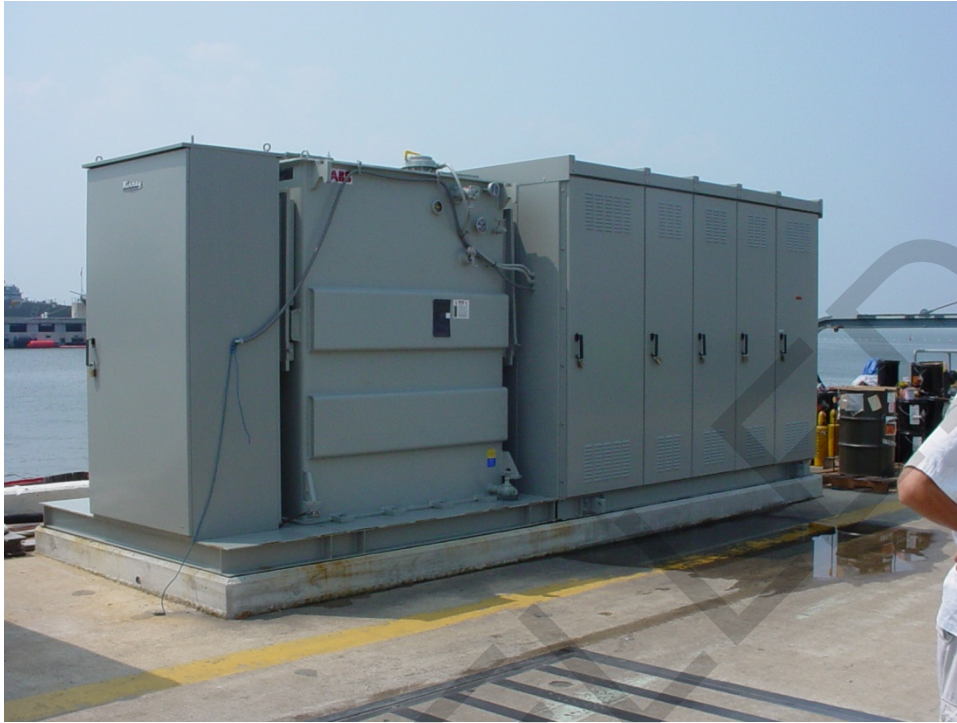
Figure 12-5. Skid-Mounted Substation with Single-Pole Connections
