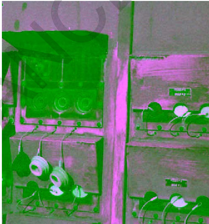
Figure 12-5. Skid-Mounted Substation with Single-Pole Connections
