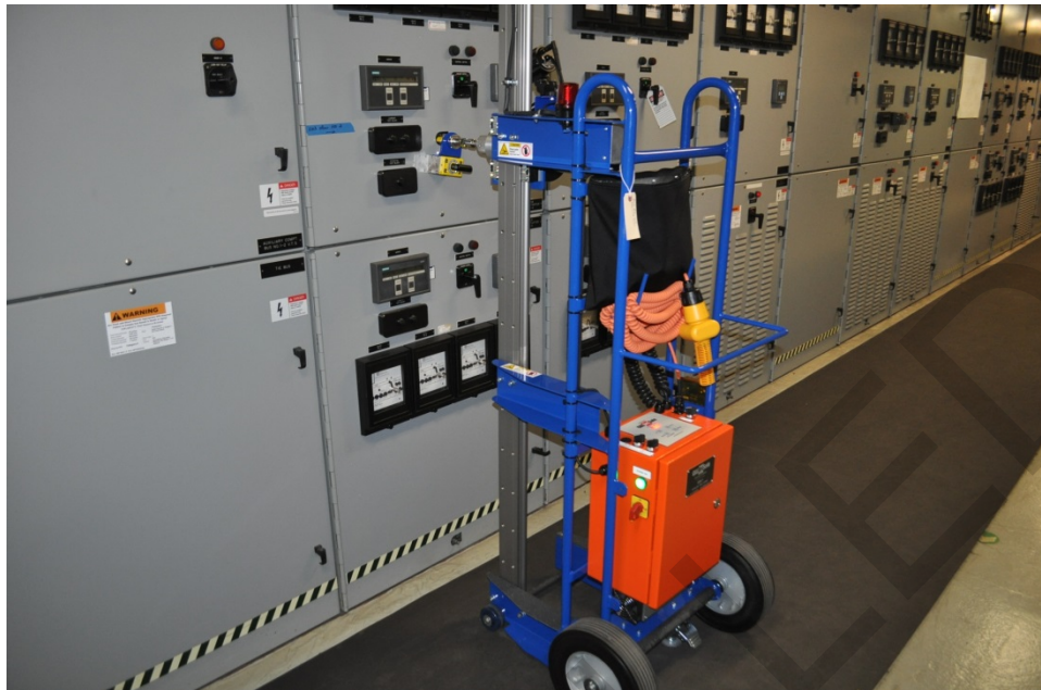
Figure 1. Remote Racking Mechanism
