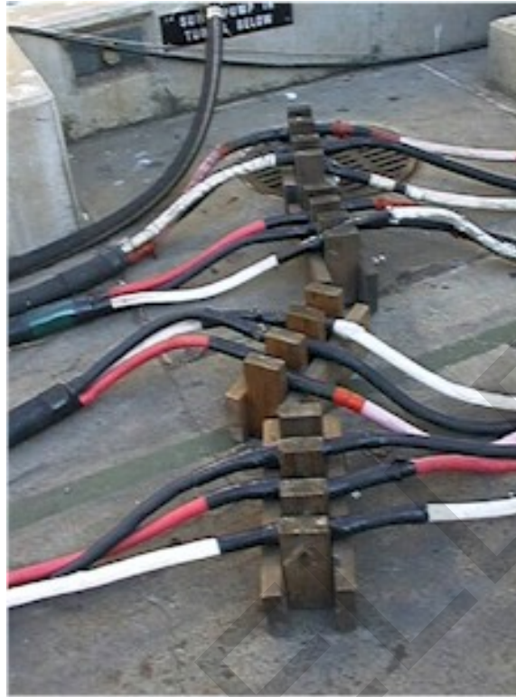
Figure 12-13. 480 Volt Shore-Cable to Ship-Cable Splice Connection in Place
