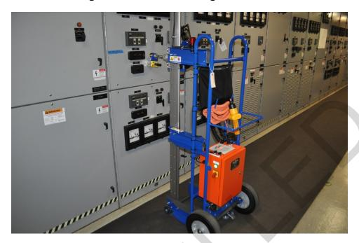
Figure 1. Remote Racking Mechanism
