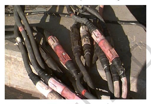
Figure 12-12. 480 Volt Shore-Cable to Ship-Cable Plug and Receptacle Connection In Place
