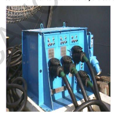
Figure 12-11. 480 Volt Shore-Cable to Ship-Cable with Single-Pole Connection
