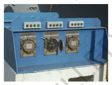
Figure 12-8. 4.16 kV Pier Electrical Outlet Assembly and Outlets – Existing Installations
