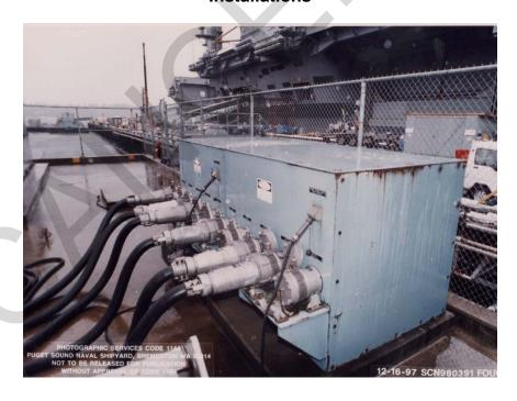
Figure 12-9. 4.16 kV Pier Electrical Outlet Assembly and Outlets – Newer Designs
