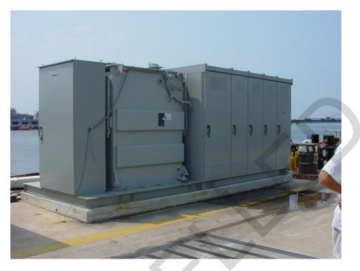
Figure 12-5. Skid-Mounted Substation with Single-Pole Connections
