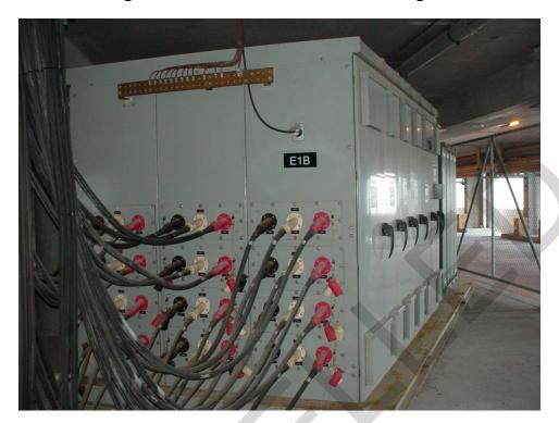
Figure 12-6. Double-Deck Pier Switchgear
