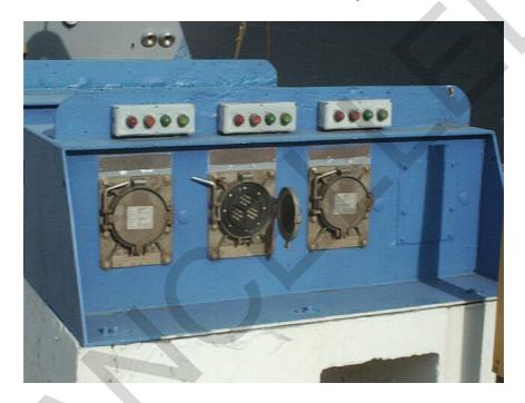
Figure 13-7. 480 Volt Pier Electrical Outlet Assembly Without Cable Connections
