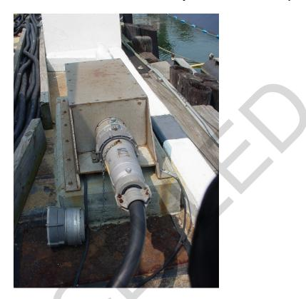
Figure 13-1. Electrical Connection Outlet Assembly with a 15 kV Receptacle
