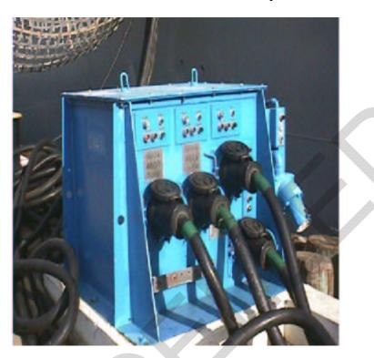
Figure 13-10. 480 Volt Pier Electrical Outlet Assembly and Cable Connections
