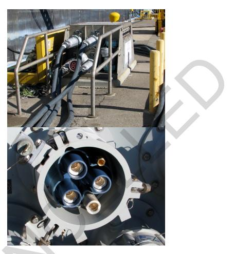
Figure 13-9. 4.16 kV Pier Electrical Outlet Assembly and Outlets – Newer Designs
