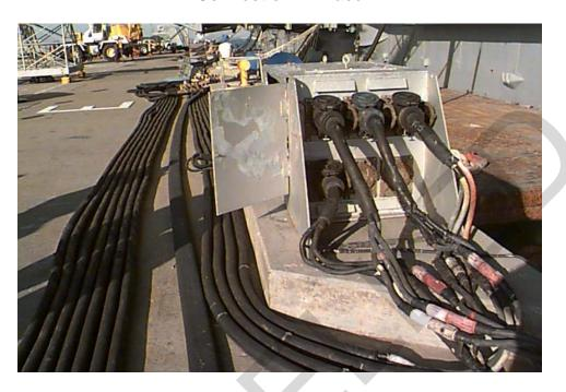
Figure 13-13. 480 Volt Shore-Cable to Ship-Cable Splice Connection in Place
