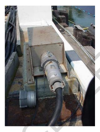
Figure 13-2. Close-Up of Electrical Connection Outlet Assembly
