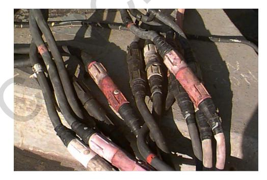
Figure 13-12. 480 Volt Shore-Cable to Ship-Cable Plug and Receptacle Connection In Place
