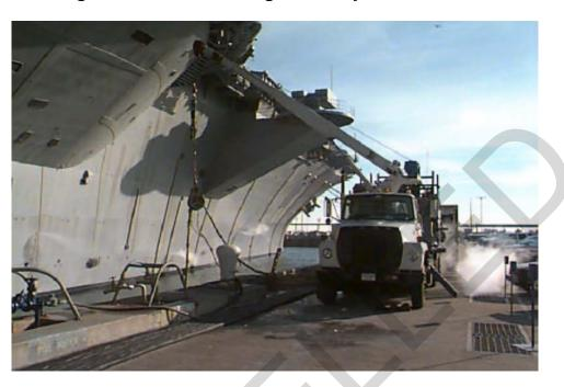
Figure 13-17. Cable Being Reeled by a Boom Truck.
