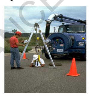
Figure 14-6. Vault/Manhole Rescue
