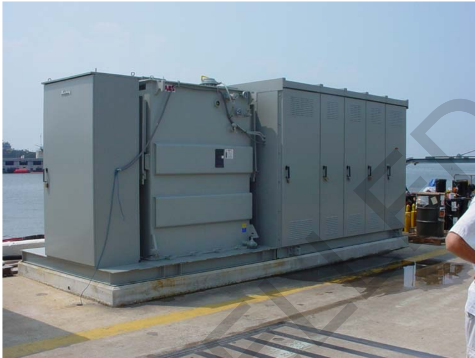
Figure 13-5. Skid-Mounted Substation with Single-Pole Connections
