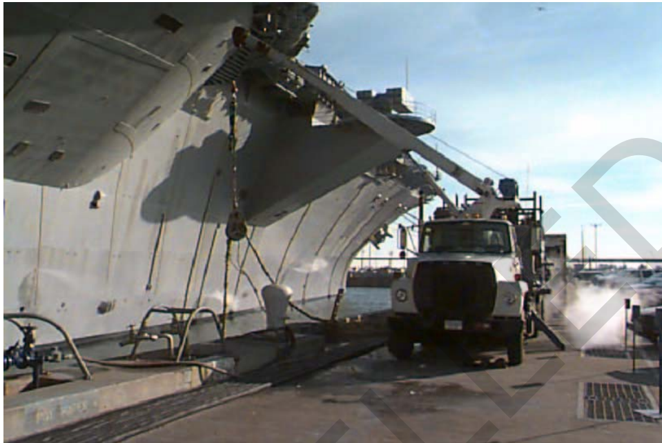
Figure 13-16. Cable Being Reeled by a Boom Truck.
