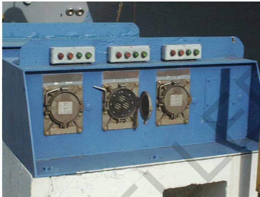
Figure 13-8. 4.16 kV Pier Electrical Outlet Assembly and Outlets
