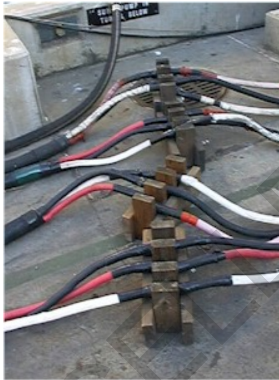
Figure 13-12. 480 Volt Shore-Cable to Ship-Cable Splice Connection in Place
