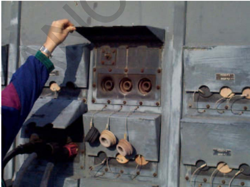
Figure 13-5. Skid-Mounted Substation with Single-Pole Connections
