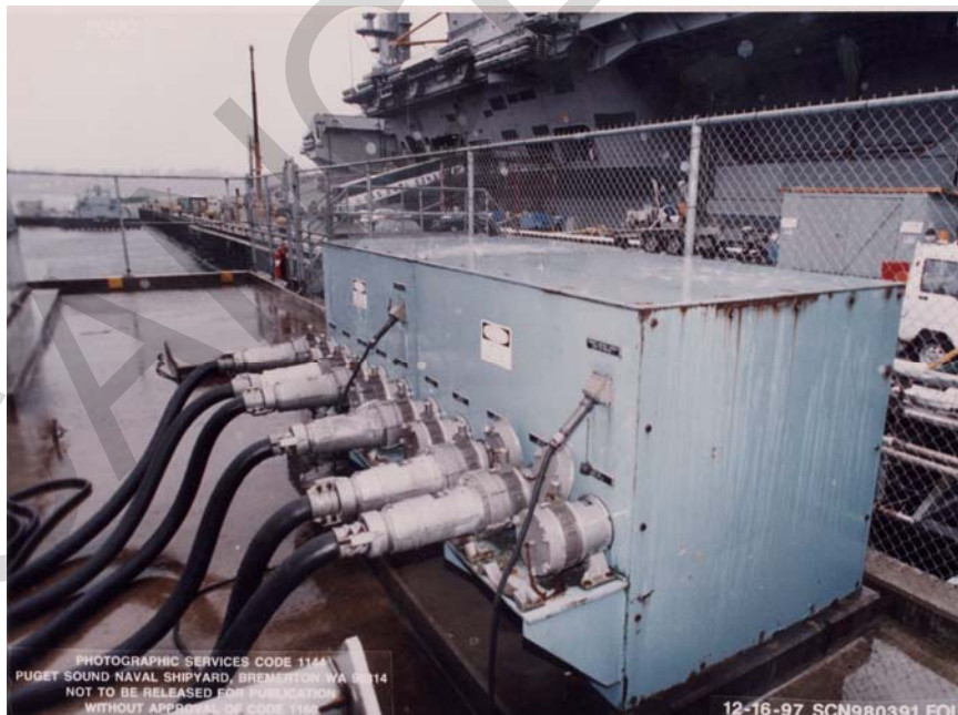
Figure 13-8. 4.16 kV Pier Electrical Outlet Assembly and Outlets
