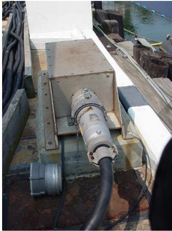
Figure 13-2. Close-Up of Electrical Connection Outlet Assembly
