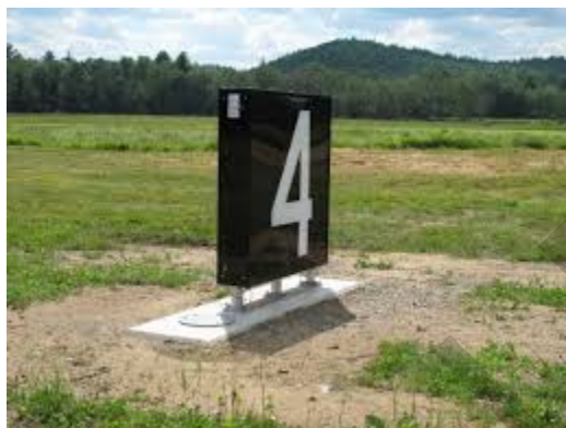
Figure 13-17 Runway Distance Remaining Sign (Lighted)
