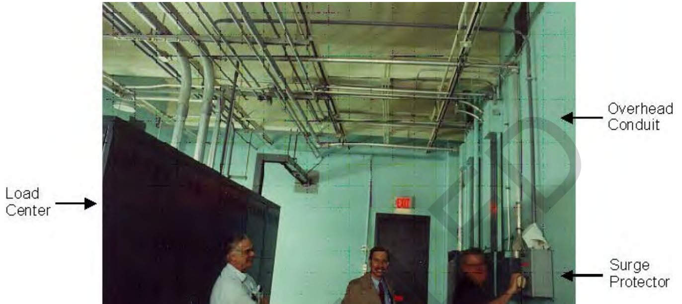
Figure 11-5. Less-Than-Optimal Installation by Including Safety Switch
