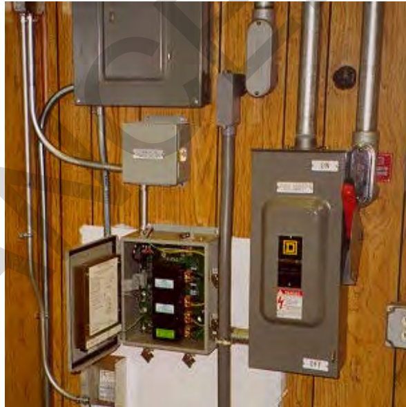
Figure 11-5. Less-Than-Optimal Installation by Including Safety Switch
