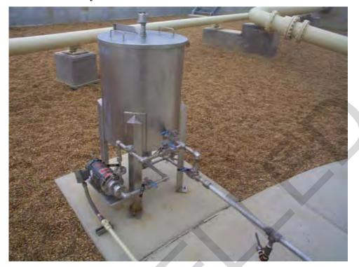
Figure 7.3. Water Draw-Off System Detail.
