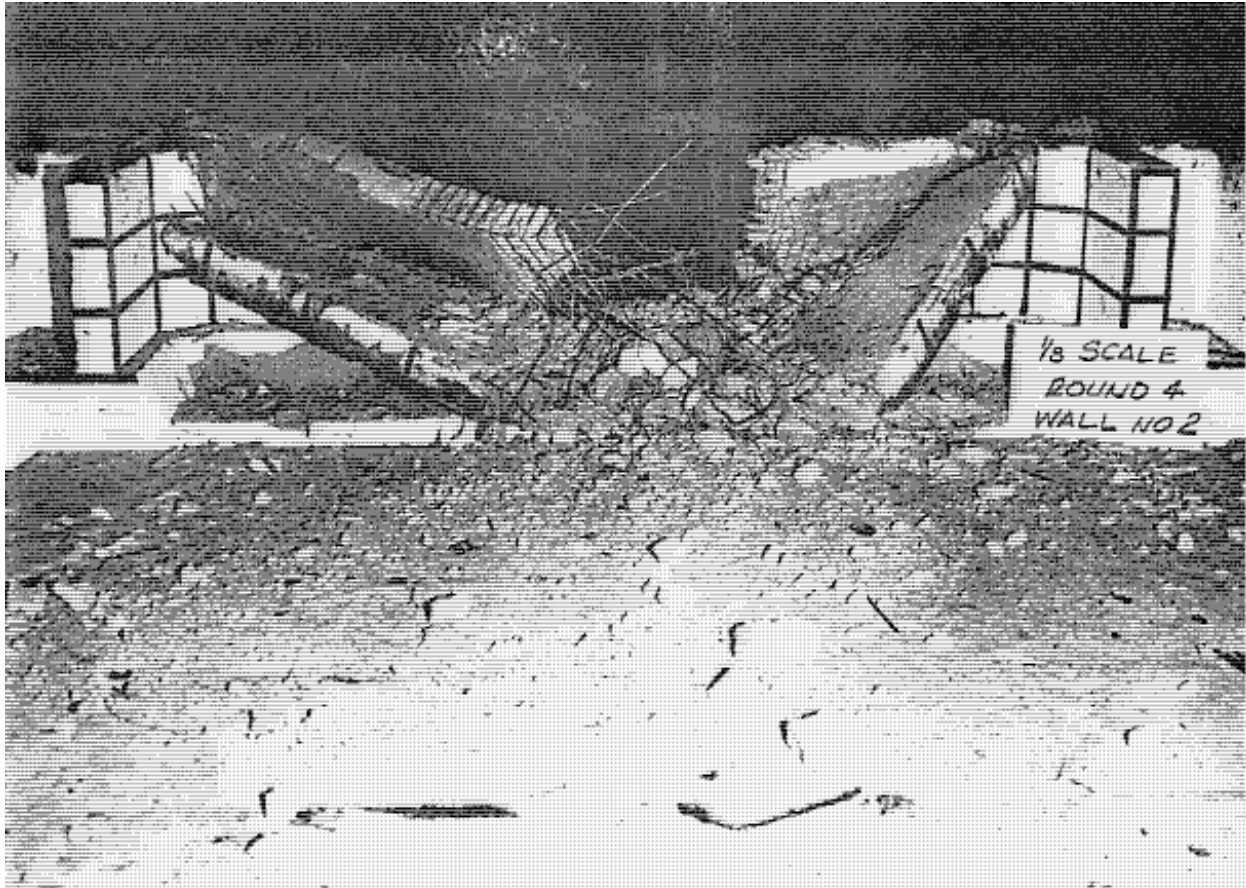
Figure 4-71 Backwall Failure of Cubicle with Laced Reinforcement
