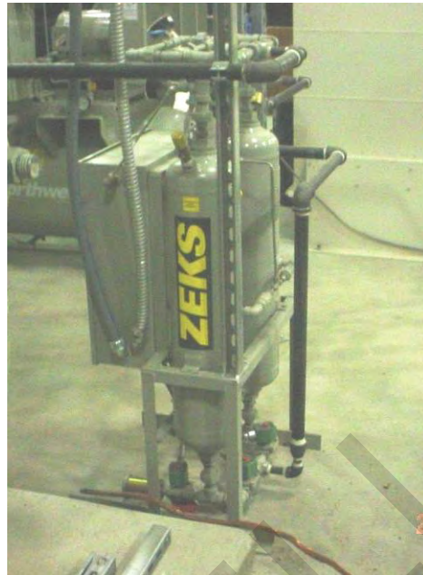
Figure 3.7. Desiccant Air Dryer Assembly
