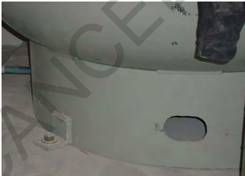
Figure 3.9. Air Receiver Tank Load Path
