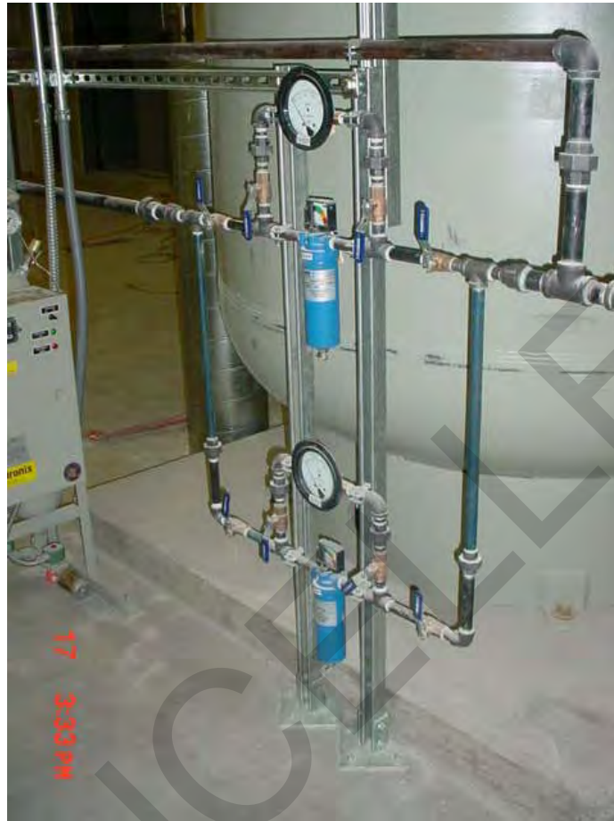
Figure 3.8. Coalescing Air Filters are Line-Mounted
