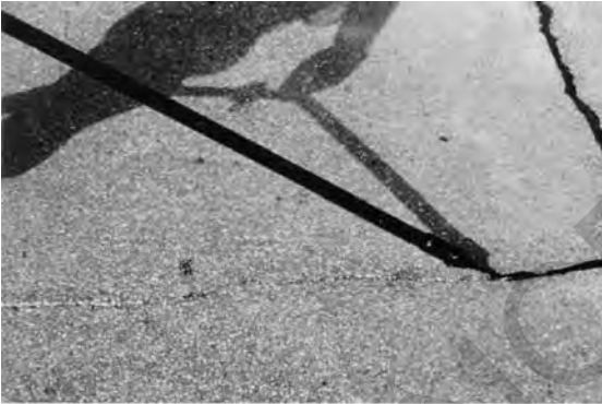
Figure 9.3. Sealing the crack
