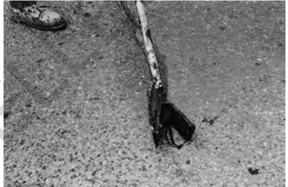
Figure 9.4. Using a squeegee to remove excess sealant
