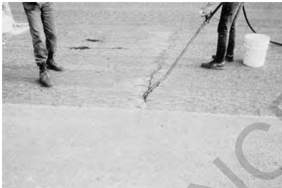
Figure 9.1. Filling crack with sand emulsion mixture
