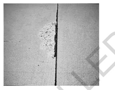
Figure 13-2 Incompressible Causing Spalling at a Joint or Crack
