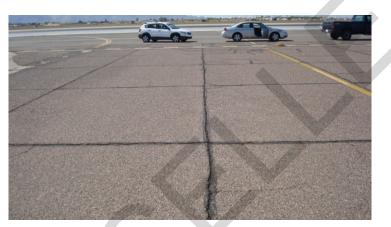
Figure 9-2 Reflective Cracking
