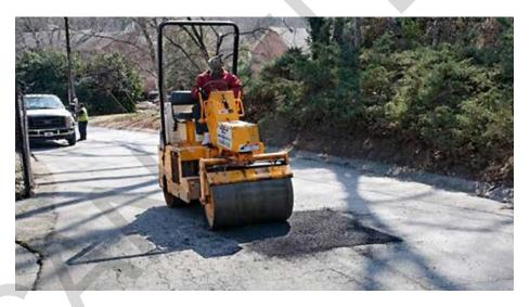
Figure 3-9 Check Level of Patch Surface
