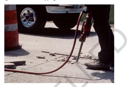
Figure 18-5 Use of Chipping Hammers to Remove Concrete
