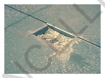
Figure 13-8 Compressible Insert
