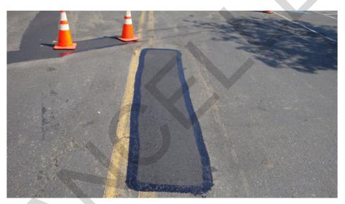
Figure 3-10 Seal the Edges
