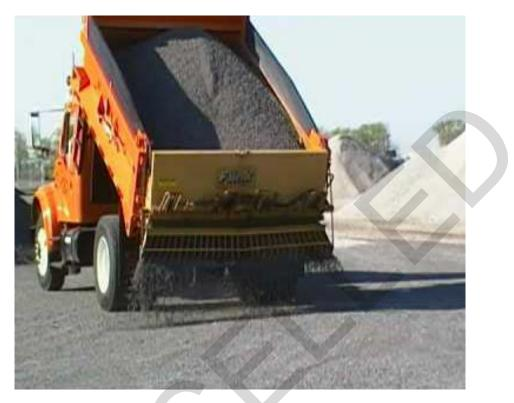
Figure 6-1 Applying Aggregate with Tailgate Spreader on Dump Truck
