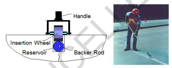
Figure 2-1 Installation of Backer Rod
