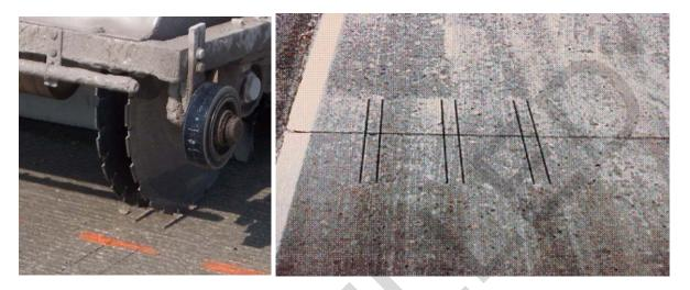
Figure 18-2 Gang-Mounted Multiple Saw Blades for Slot Cuts
