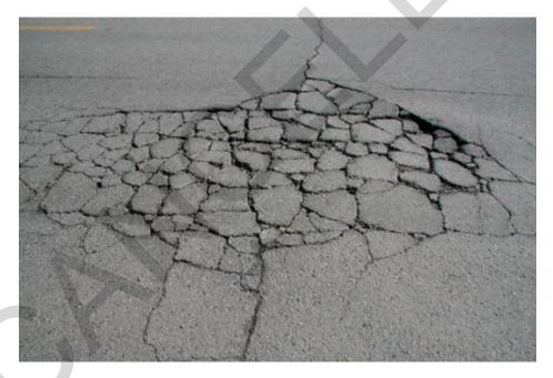
Figure 9-1 Alligator Cracking
