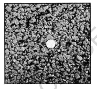
Figure 8.1. View of a porous friction surface (PFS)
