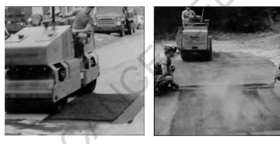
Figure 3.13. Sealing edges of the patch
