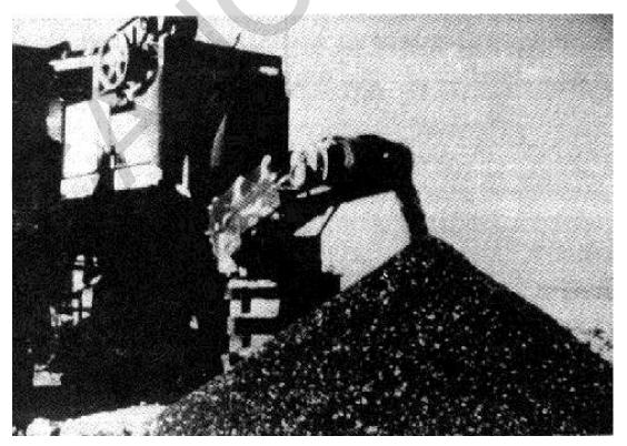
Figure 3-3. Old asphalt concrete pavement after crushing.
