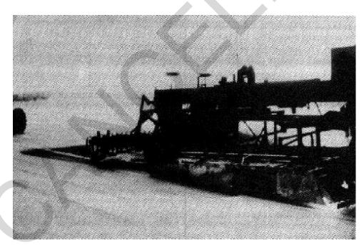
Figure 2-4. Heater with scarifying teeth followed by grader.
