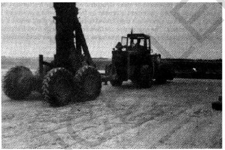
Figure 5-2. Diesel pile-driving hammer puncturing the old pavement.
