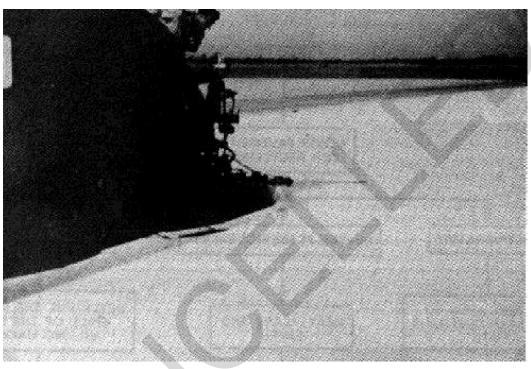
Figure 2-2. Asphalt distributor applying rejuvenator.
