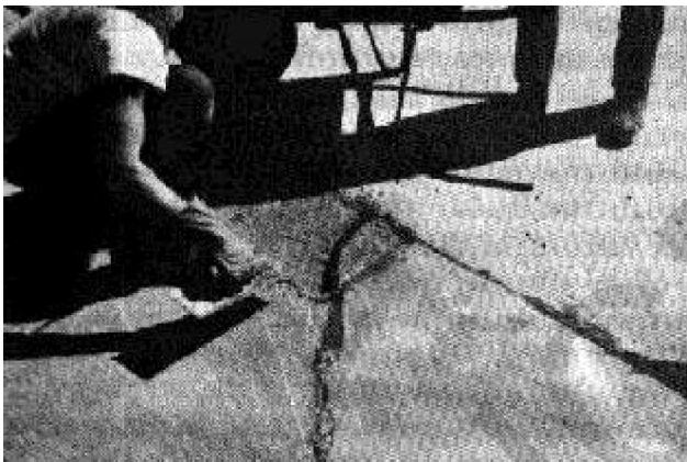
Figure 4. Finishing a patch containing an active crack.
