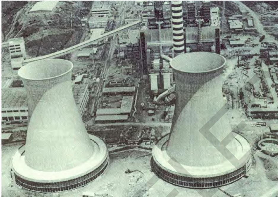
Figure 4-5. Hyperbolic Natural-Draft Cooling Towers
