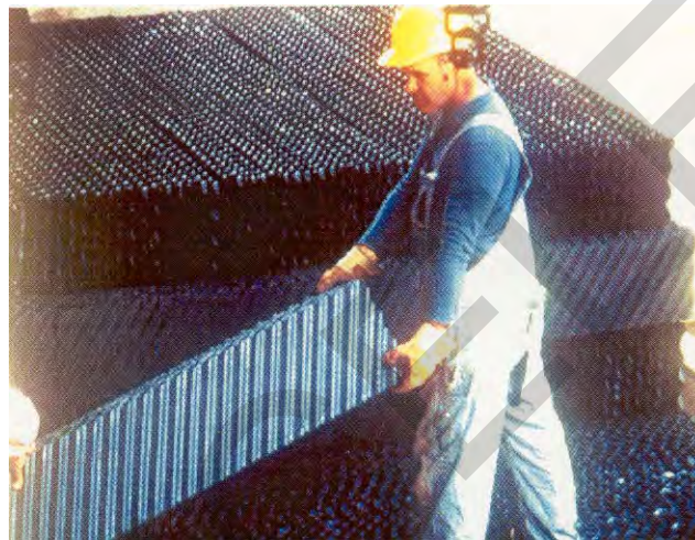
Figure 4-11. High-Efficiency Cooling Tower Film Fill
