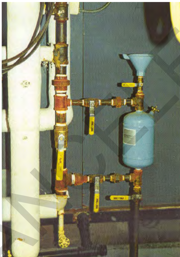
Figure 7-1. Chemical Pot Feeder
