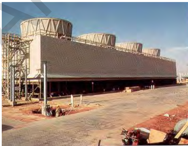
Figure 4-9. Counter-Flow Cooling Tower
