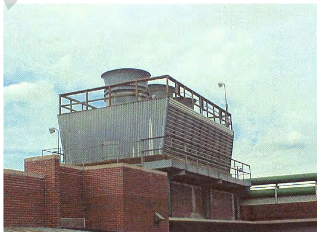
Figure 4-7. Cross-Flow Cooling Tower
