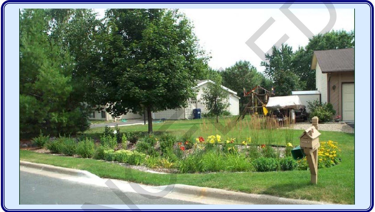
Figure B-1 Typical Bio-infiltration ‘Rain Garden’
