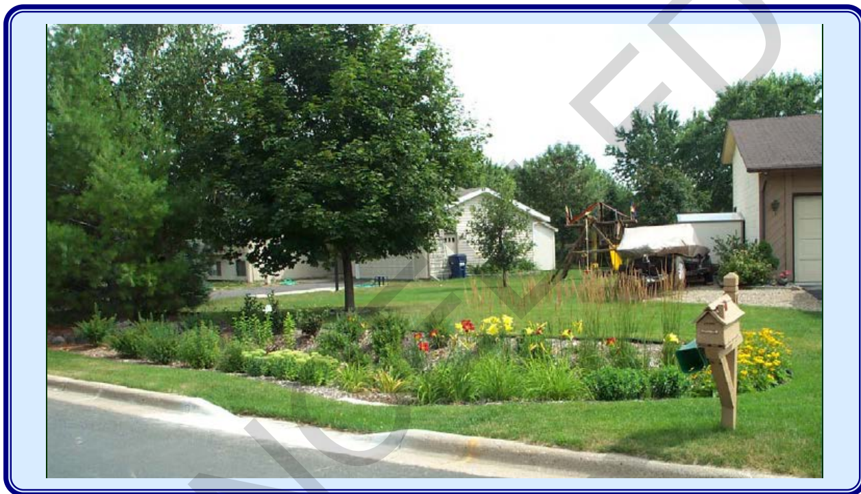
Figure B-1 Typical Bio-infiltration ‘Rain Garden’
