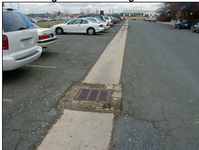
Figure 10-2. Drainage Inlet
