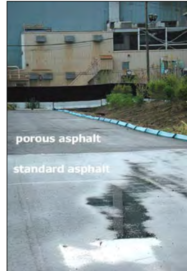
Figure 8-15. Drainage in Both Types of Pavement
