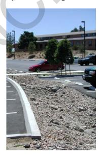
Reducing the size of parking lots is ultimately the best way to minimize negative effects of impervious surfaces. Scrutinize the parking requirements; parking lots may not need to be designed for peak use. Overflow parking areas constructed of pervious materials may meet the occasional peak demand, reducing stormwater runoff and increasing on-site infiltration.
