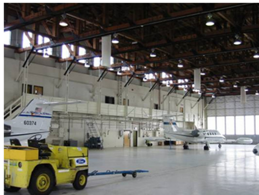
Figure A-7 Example of Clerestory Application
