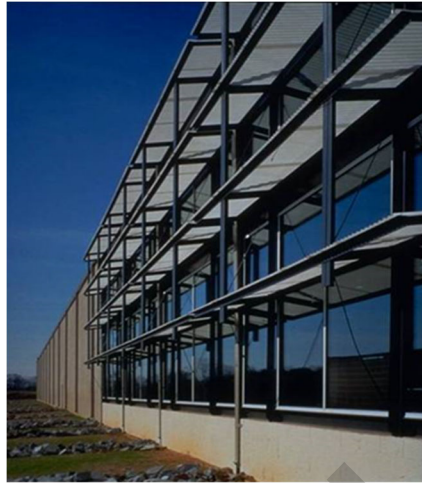
Figure A-4 Example of Architectural Shading Devices
