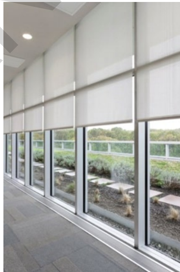
Figure A-12 Example of Solar-Adaptive Shading
