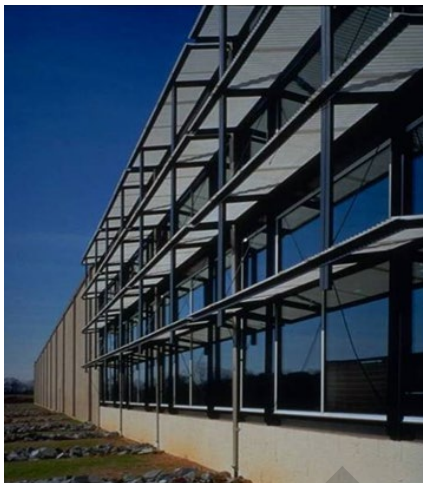
Figure A-4 Example of Architectural Shading Devices
