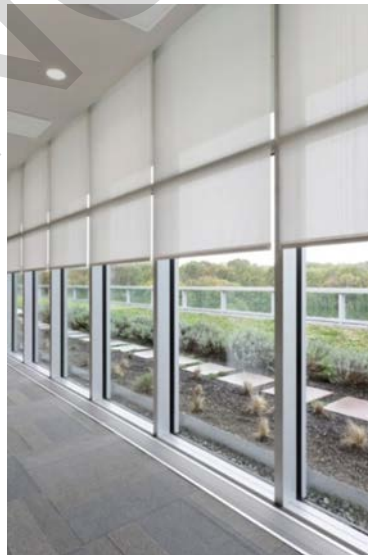
Figure A-12 Example of Solar-Adaptive Shading
