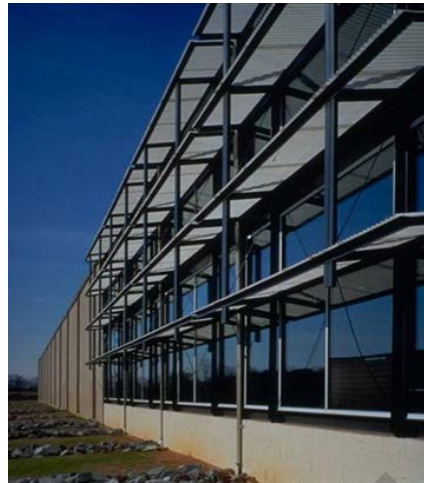
Figure A-4 Example of Architectural Shading Devices
