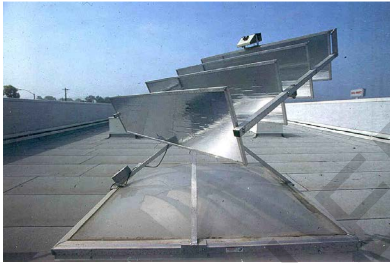
Figure A-11 Example of an Active Daylighting System that Tracks the Sun and Directs Daylight into the Building
