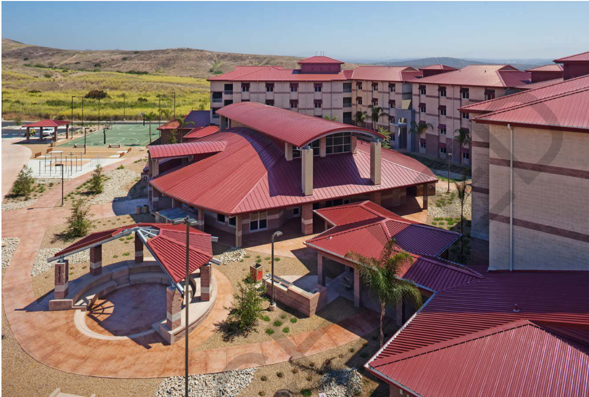
Figure B-4 Best Practice, BEQ Campus Sun shading and Walkways
