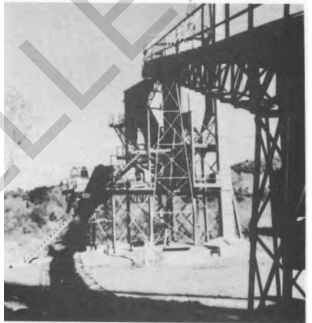
Figure 4-5. Batch-type central plant used for mixing soil-cement.
