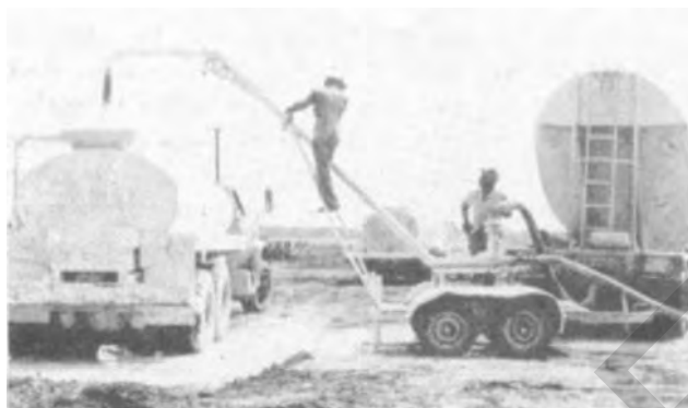
Figure 4-30. Jet slurry mixing plant.
