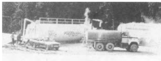
Figure 4-34. Portabatch lime slaker.
