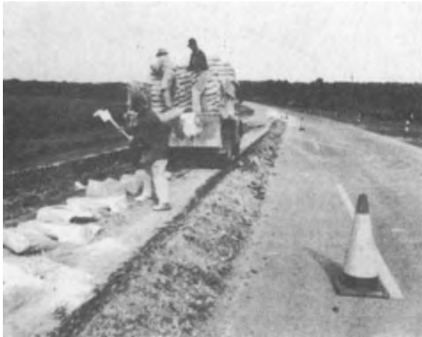
Figure 4-24. Application of lime by the bag for a small maintenance project.
