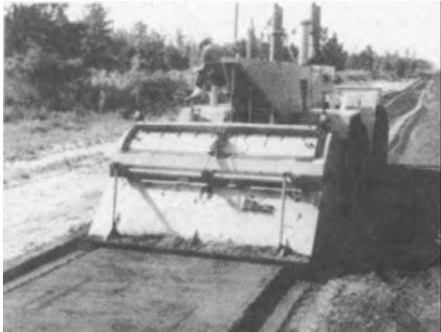
Figure 4-49. Single-shaft rotary mixer without asphalt.
