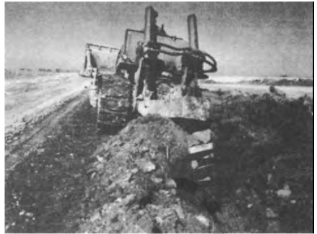
Figure 4-17. Deep stabilization after lime spreading the plow cuts 24 inches deep.
