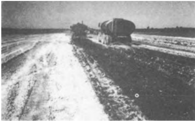
Figure 4-35. Watering of lime-treated clay on airport project.
