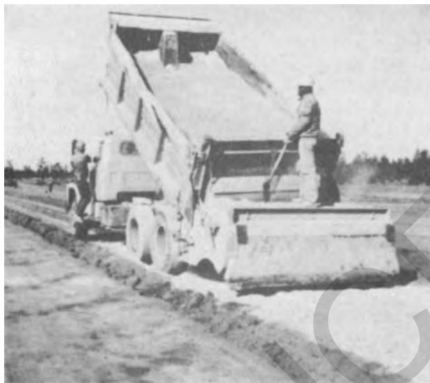
Figure 4-8. Mechanical cement spreader attached to a job dump truck spreading cement in regulated quantities.
