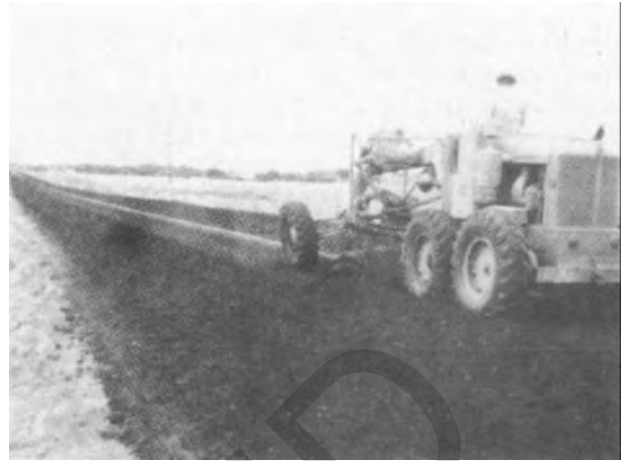
Figure 4-50. Mixing with motor grader.
