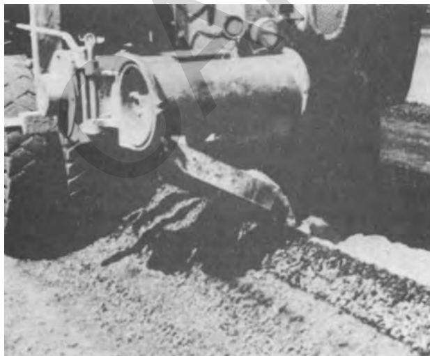
Figure 4-9. Windrow-type mechanical spreader placing cement on windrow.
