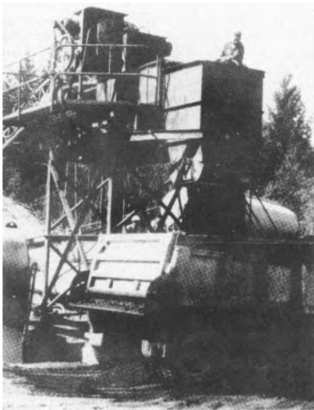
Figure 4-53. Stationary cold-mix plant.
