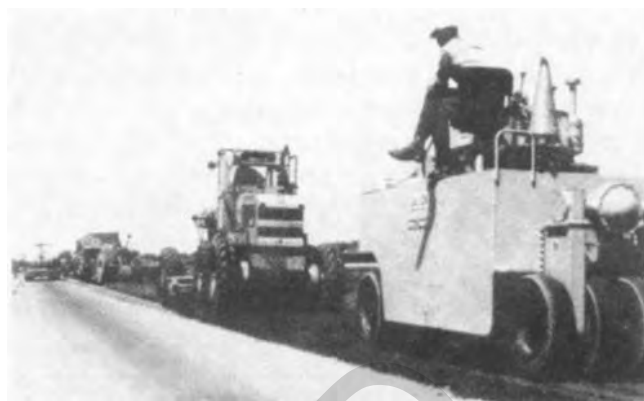
Figure 4-52. Spreading and compacting train.
