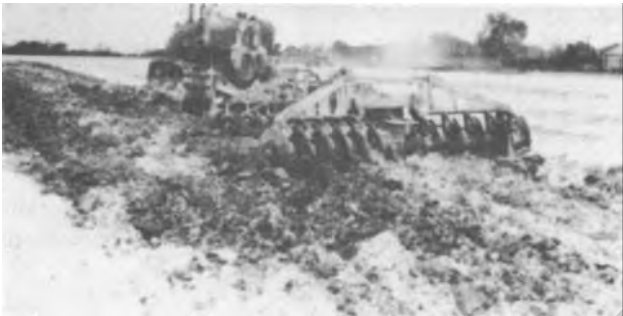
Figure 4-36. Mixing with a disc harrow.
