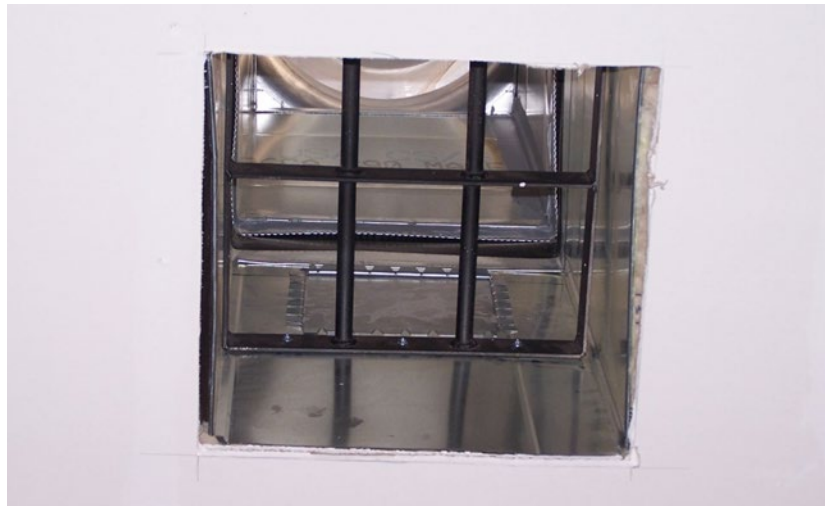
Figure 3-13 Bars on Penetration
