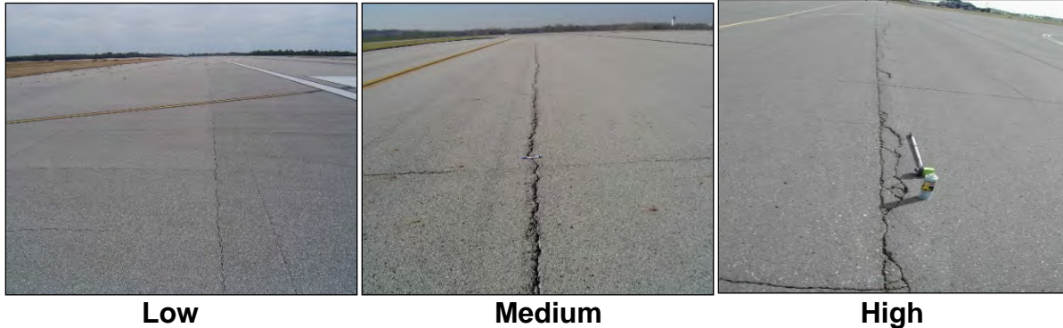
Figure B-7 Joint Reflection Cracking Severity Levels
