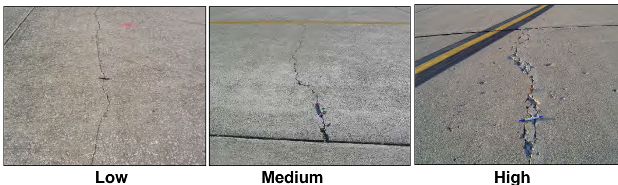
Figure C-3 Longitudinal, Transverse, and Diagonal Cracks Severity Levels
