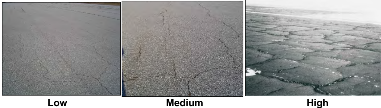
Figure B-3 Block Cracking Severity Levels
