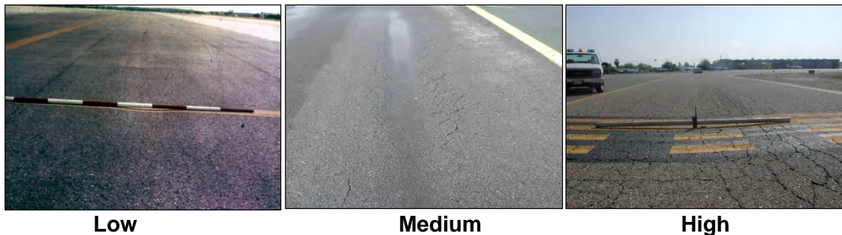
Figure B-16 Rutting Severity Levels
