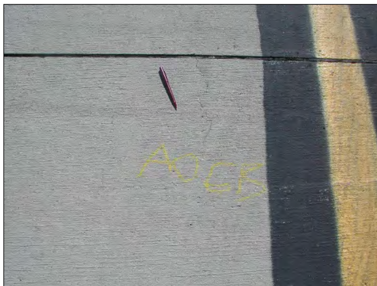
Figure C-14 Shrinkage Cracks
