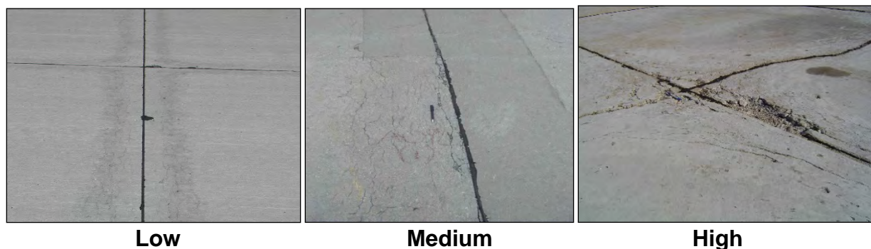
Figure C-5 Durability “D” Cracking Severity Levels
