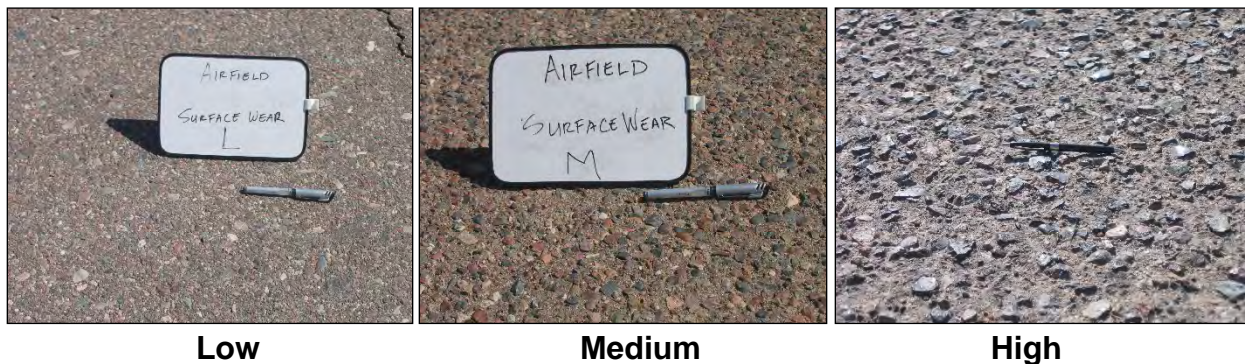
Figure B-20 Weathering Severity Levels
