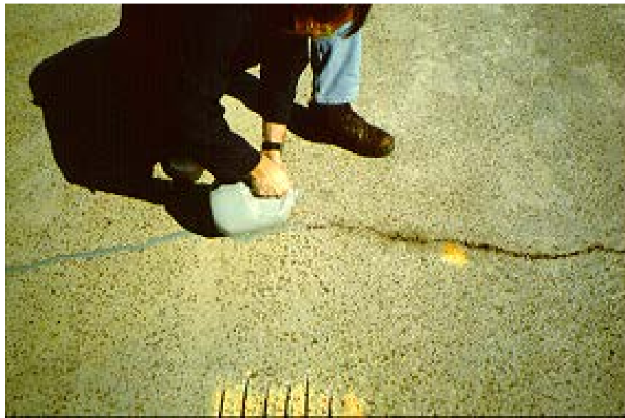
Figure 2-5 Applying Modified Grout to Seal RMP Crack
