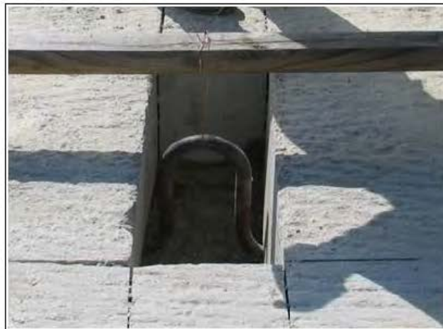
Figure 13. Hat-Type Tie-Down Prior to Concrete Placement.
