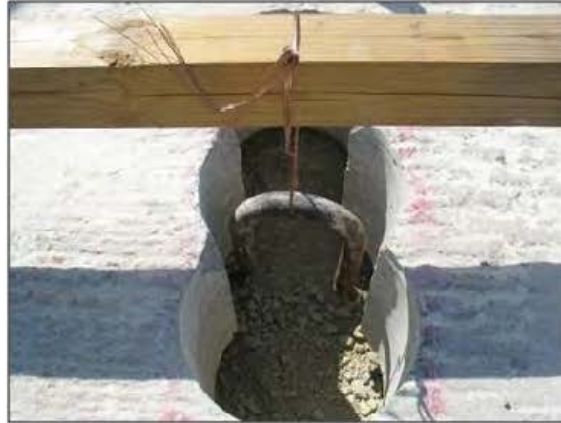
Figure 19. Hat-Type Tie-Down Installed Using Coring Method Prior to PCC Placement.
