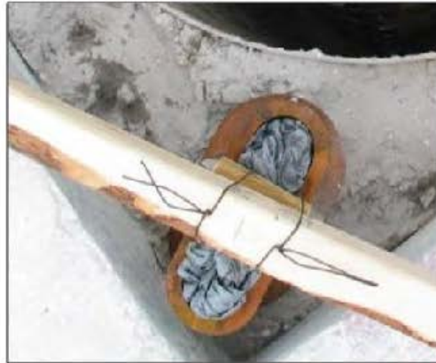
Figure 6. Neenah Anchor Bowl Filled With a Rag.
