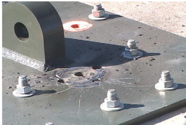
Figure 12. Anchor Plate with Bolts, Nuts and Washers in Place
