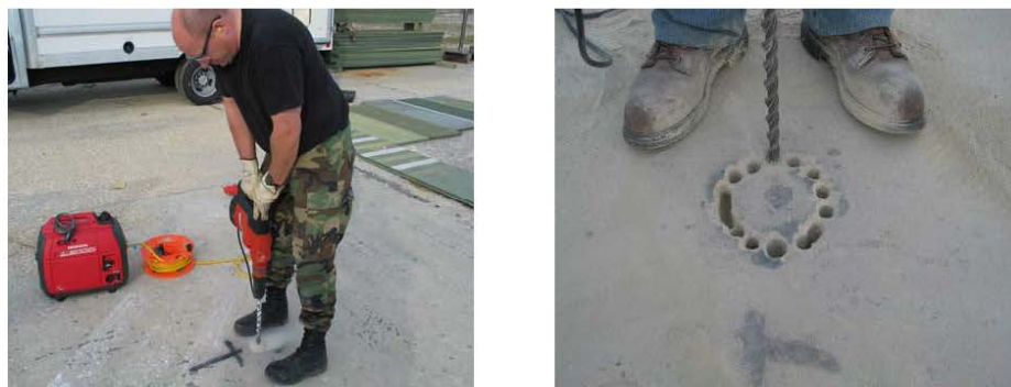
Figure 8. Drilling Anchor Hole Perimeter
