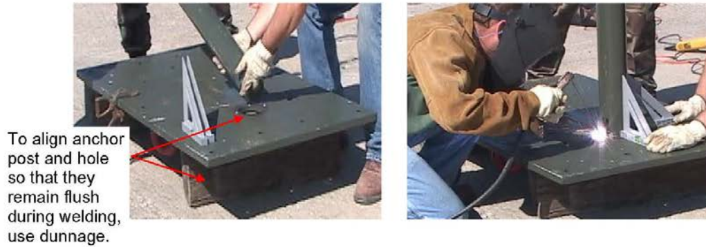
Figure 10. Welding Anchor Post to Anchor Plate
