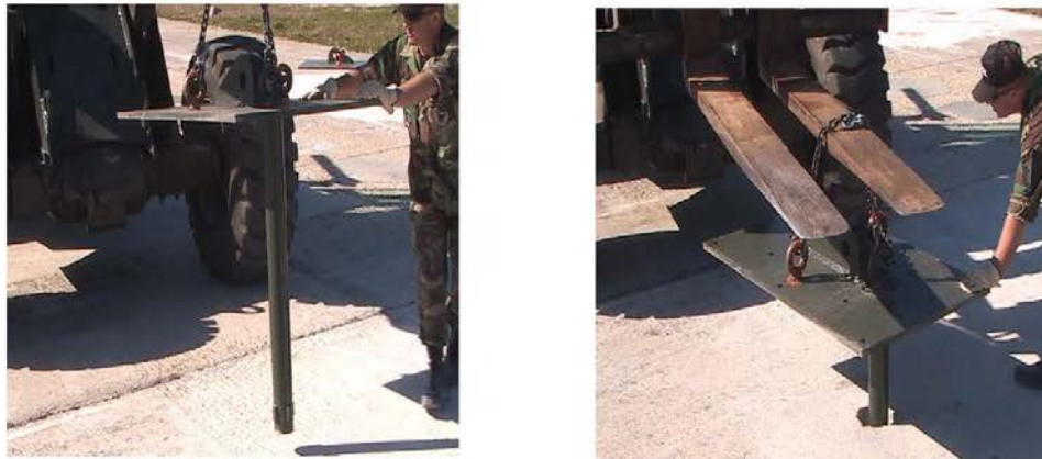
Figure 11. Lowering the Expedient Anchor Plate into the Hole
