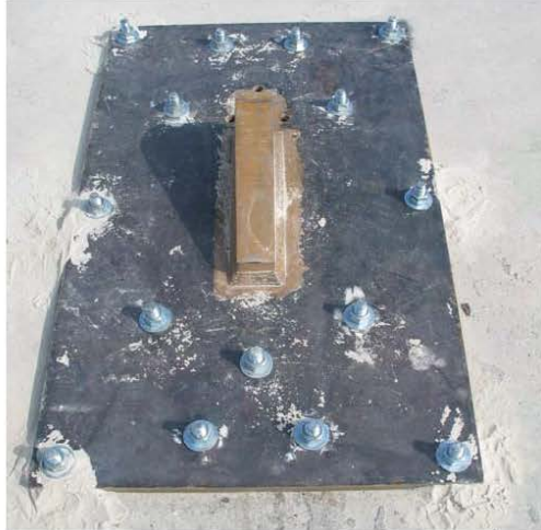
Figure 14. Completed Anchor Plate
