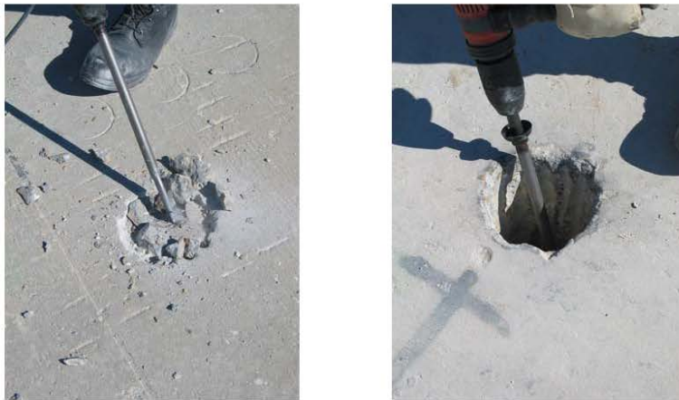
Figure 9. Chiseling Anchor Hole
