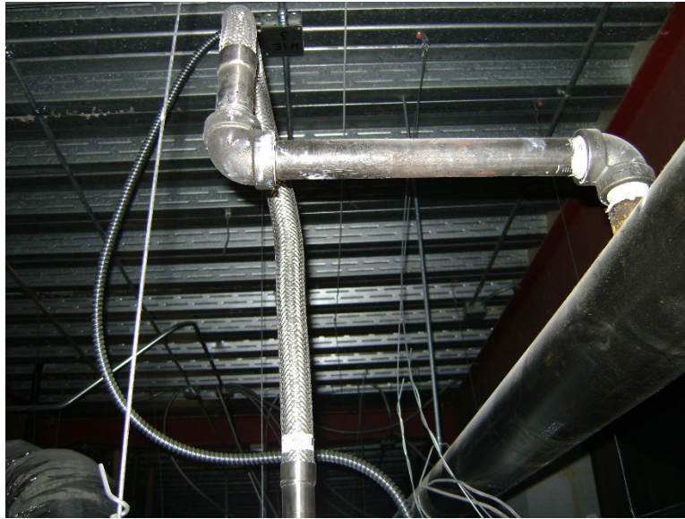
Figure 4-7 Example Flexible Sprinkler Hose Fitting (Courtesy of TERPconsulting)
