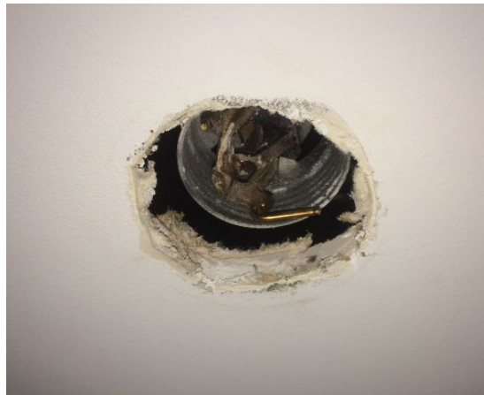
Figure 3-10 Concealed Sprinkler Damaged by Earthquake (Courtesy of Accel Fire Protection)
