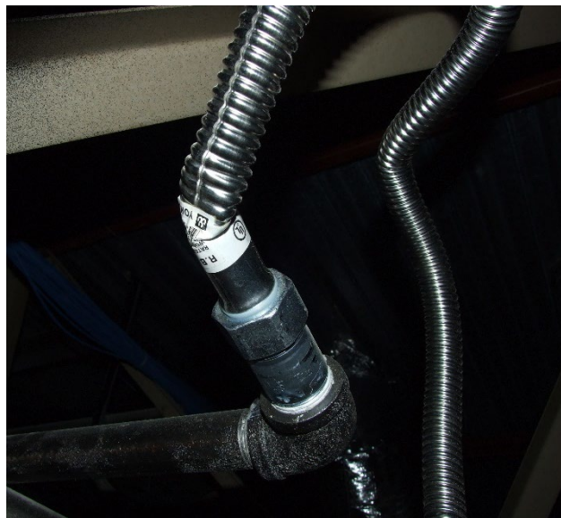
Figure 5-3 Kink in Flexible Hose (Courtesy of Ralph K. Foster, III, PE, FSFPE)
