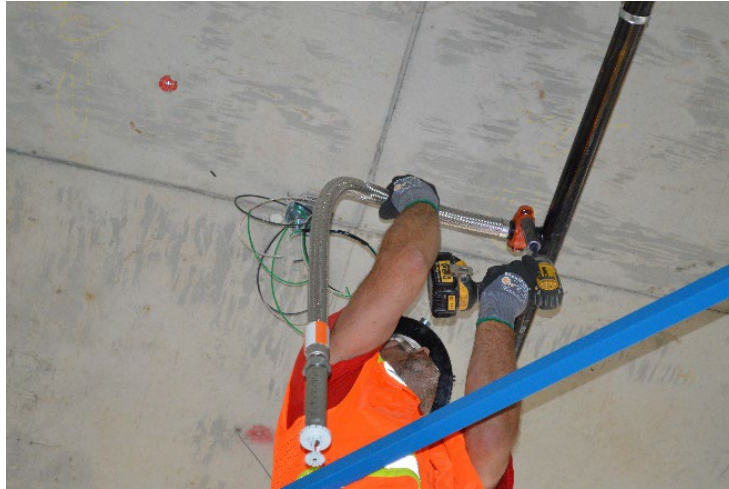
Figure 5-2 Installation of Flexible Hose Fitting with Grooved Branch Line Adapter (Courtesy of Victaulic)
