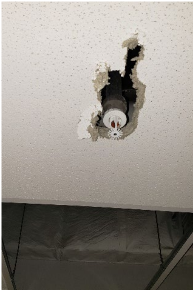
Figure 3-10 Concealed Sprinkler Damaged by Earthquake (Courtesy of Accel Fire Protection)
