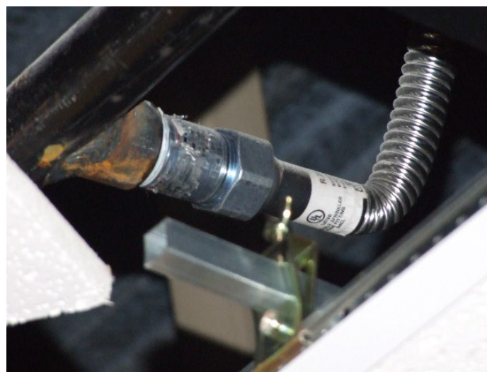
Figure 4-8 Kink or Shallow Bend in Flexible Hose (Courtesy of Ralph K. Foster, III, PE, FSFPE)
