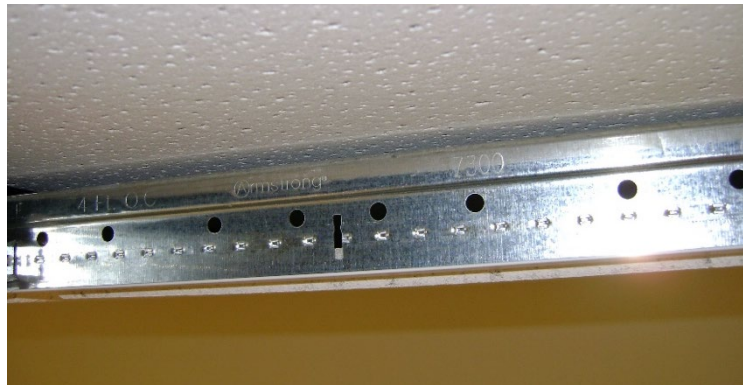
Figure 4-4 Ceiling Grid with Manufacturer's Label (Courtesy of TERPconsulting)
