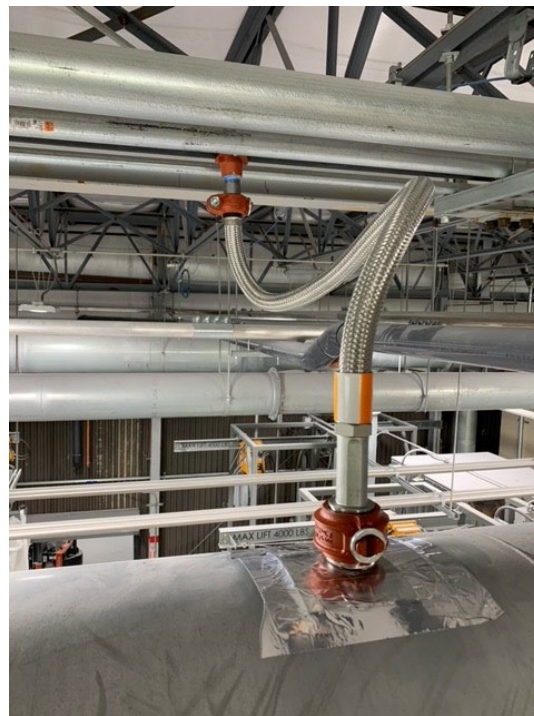
Figure 3-4 Industrial Duct Sprinkler Installation on Round Duct (Courtesy of Victaulic)
