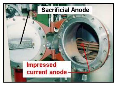
Figure 39 Impressed Current CP System for an Industrial Hot Water Storage Tank Interior, with Separate Galvanic Anode for the Electrically Isolated Manway Cover.
