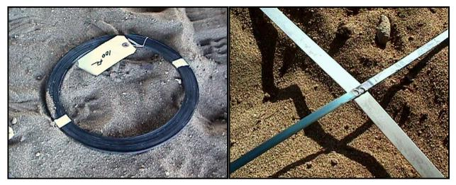
Figure 7 Roll of MMO Ribbon Anode (left). MMO Ribbon installed (right). Thinner metal strip is the MMO anode.
