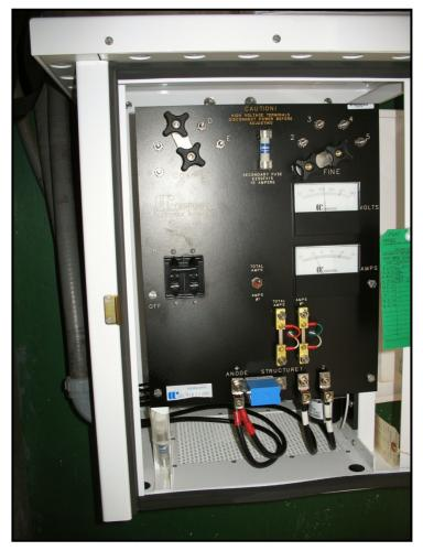
Figure 20 Typical Air-cooled Rectifier.
