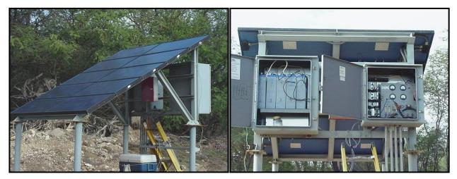
Figure 11 Solar powered CP system. Solar panels shown in picture on the left. Battery bank and control center shown in picture on the right.
