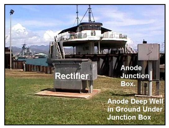
Figure 31 Deep Well Anode Impressed Current CP for Steel Sheet Pile Bulkhead
