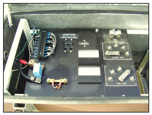
Figure 22 Typical oil-cooled rectifier with only the stacks and transformer immersed.
