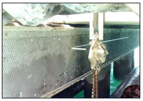
Figure 8 Mixed Metal Oxide Mesh Anode installed on a concrete beam.
