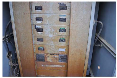
Figure 9 Severely Rusted Panelboard – 30 Years Old
