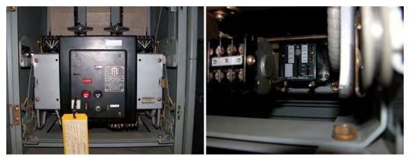
Figure 6 Low Voltage Power Circuit Breaker – 1959 Vintage Last Inspected in 1993
