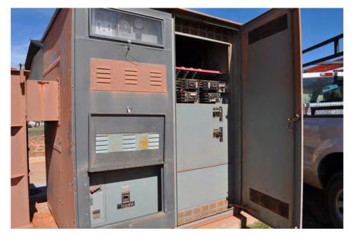
Figure 8 Outdoor Service Entrance Equipment – 25-Year Old Circuit Breakers in a Hot Environment
