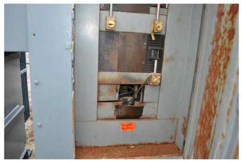
Figure 10 Deteriorated Enclosure
