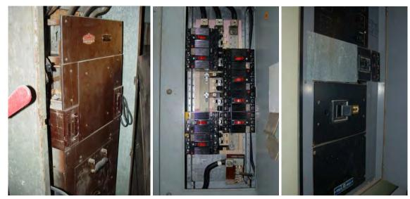
Figure 7 Old Panelboard MCCBs – Never Inspected or Tested
