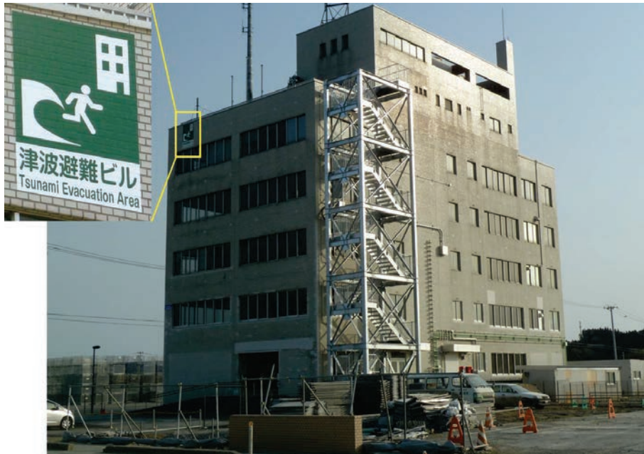
Figure 9-1 Five-story building in Kesenuma, Japan, with an exterior metal staircase installed to provide unobstructed access to the refuge area on the roof (Fraser et al., 2012).
