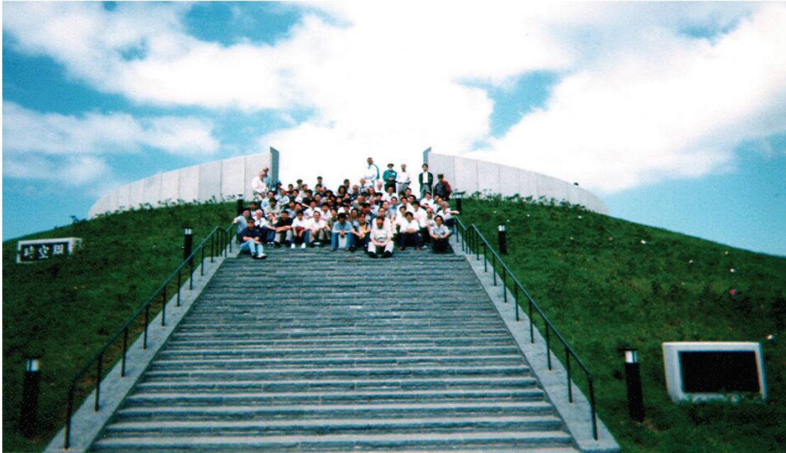
Figure A-8 Berm constructed for tsunami refuge in Aonae, Japan.
