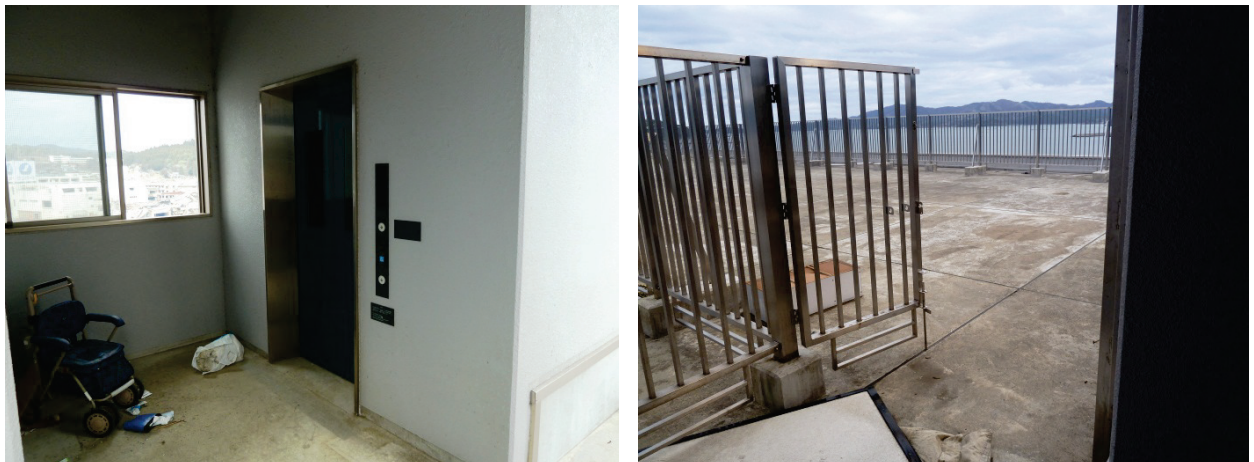
Figure 2-24 Exterior elevator and stairway access to large roof evacuation area protected by 2-meter high braced guard fence on tsunami evacuation building in Minamisanriku, Japan (photos courtesy of I. Robertson and ASCE, from Chock, et al., 2013b).
