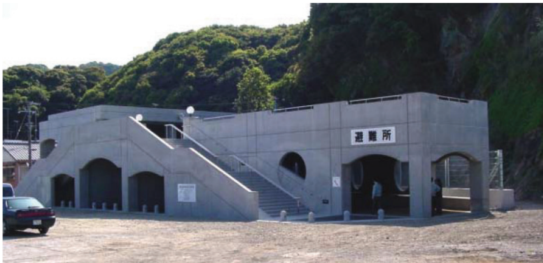
Figure A-7 Tsunami refuge in Kaifu, Japan.
