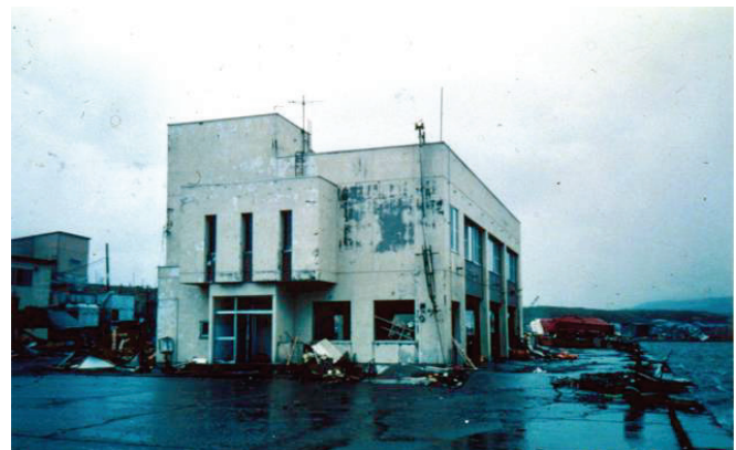
Figure 2-13 Examples of reinforced concrete structures that survived the 1993 Okushiri tsunami: vista house at Cape Inaho (left); and fish market in Aonae (right) (photo courtesy of N. Shuto).
