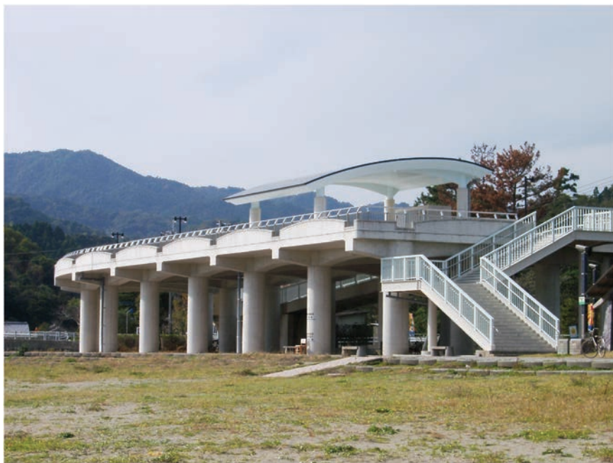
Figure 6-4 Vertical evacuation refuge structure at Shirahama Beach Resort, Japan, with limited capacity for storage of supplies (photo courtesy of N. Shuto).
