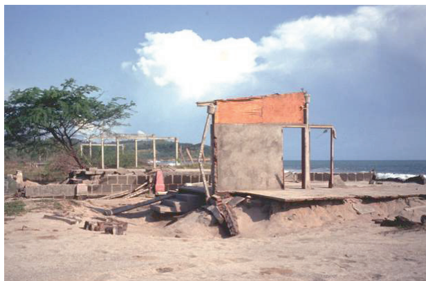
Figure 2-11 Beach houses with varying levels of damage in El Popoyo, Nicaragua, 1992 Nicaragua tsunami (photos courtesy of H. Yeh).
