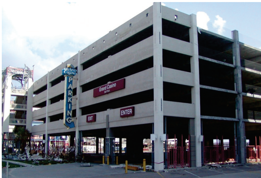
Figure 4-2 Cast-in-place reinforced concrete parking garage in Biloxi, Mississippi after Hurricane Katrina. Open structural systems allow water to pass through with minimal resistance, and interior ramps allow for easy ingress and vertical circulation.
