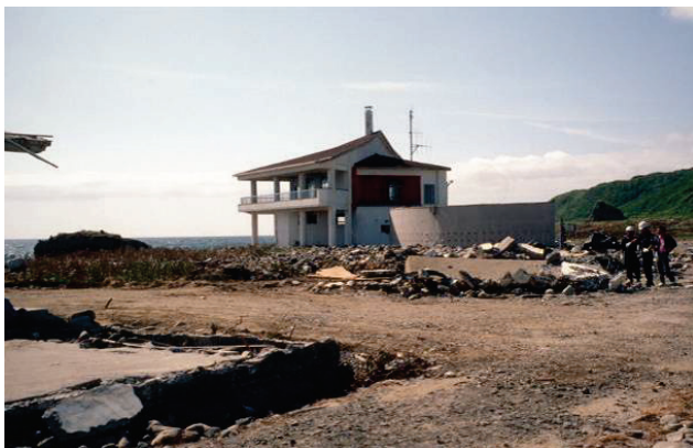
Figure 2-13 Examples of reinforced concrete structures that survived the 1993 Okushiri tsunami: vista house at Cape Inaho (left); and fish market in Aonae (right) (photo courtesy of N. Shuto).
