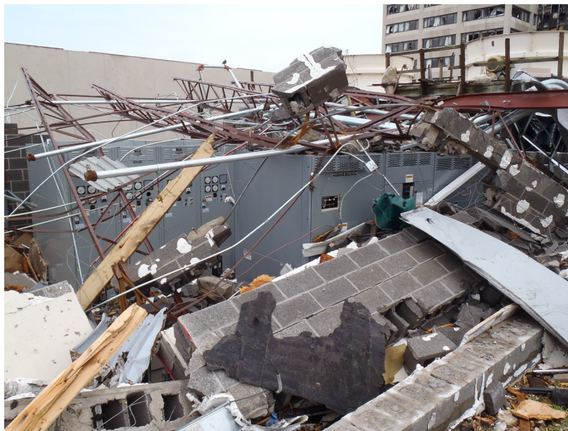
Figure 2-7 Collapsed building housing switchgear and emergency generator after the Joplin, Missouri Tornado (FEMA, 2012a).
