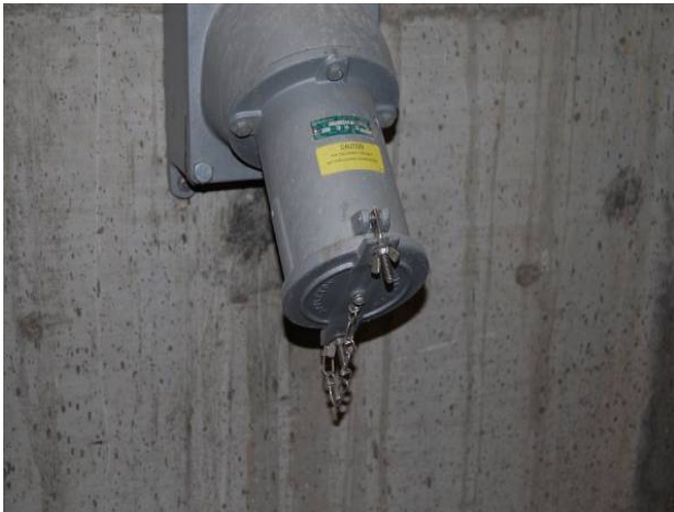
Figure 5-8 Building-mounted twist-lock plugs for connecting temporary generator cables.
