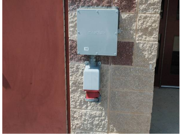
Figure 5-8 Building-mounted twist-lock plugs for connecting temporary generator cables.
