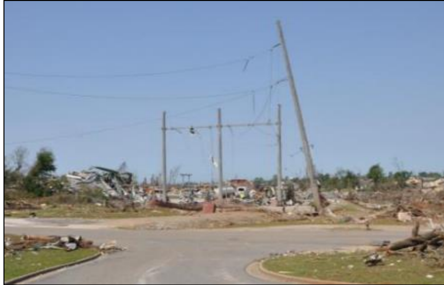
Figure 2-6 Tornado damage to transmission lines, Tuscaloosa, Alabama, April 2011 (FEMA, 2012a).
