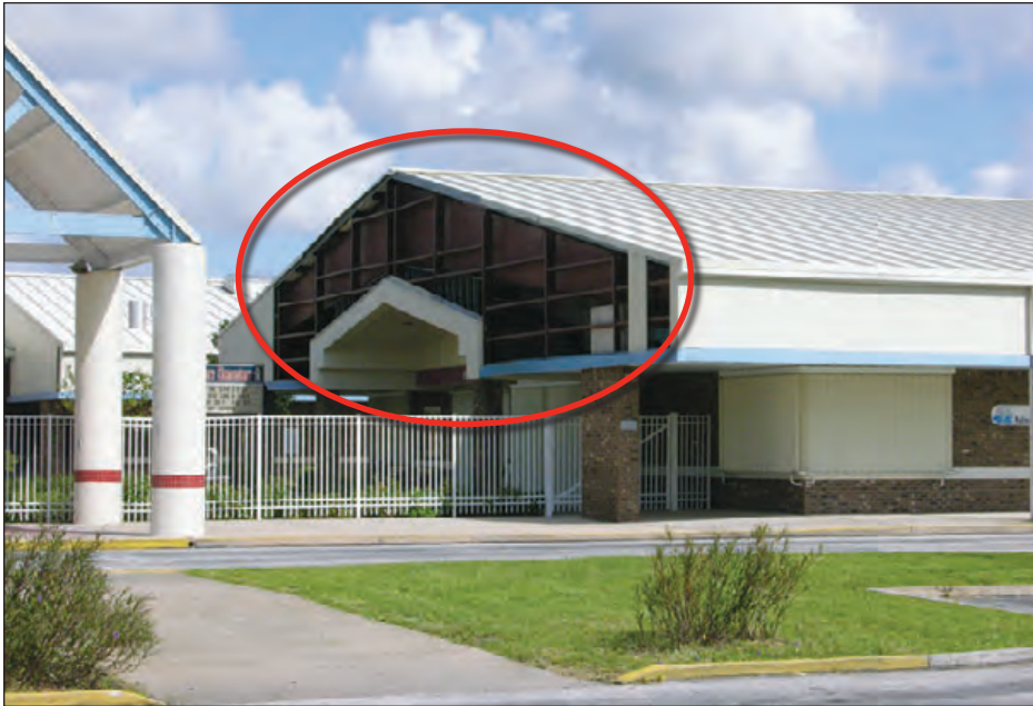
Figure 6-15: Blow-off of metal wall panels allowed wind-driven rain to enter this school. Hurricane Frances (Florida, 2004)
