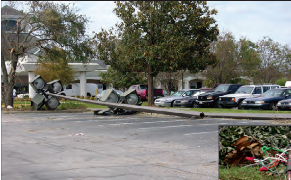
Figure 6-105: Collapsed light fixtures caused by severe corrosion (see inset). Estimated wind speed: 105–115 mph. Hurricane Ivan (Florida, 2004)
