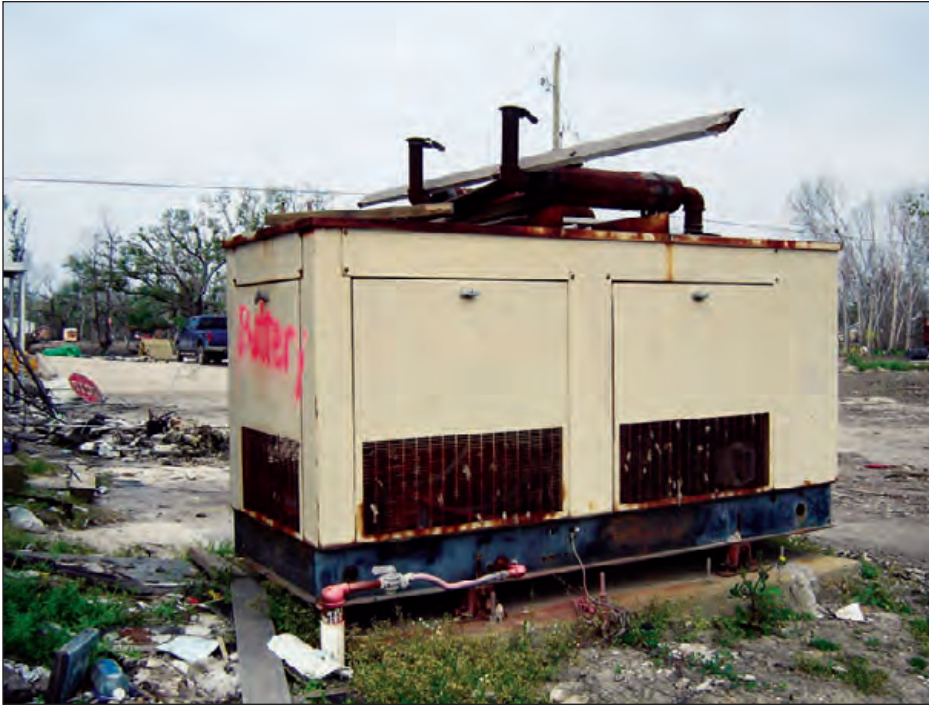
Figure 5-19: Although it was anchored and not displaced by floodwaters, this generator was out of service after being submerged (Hurricane Katrina, 2005)
