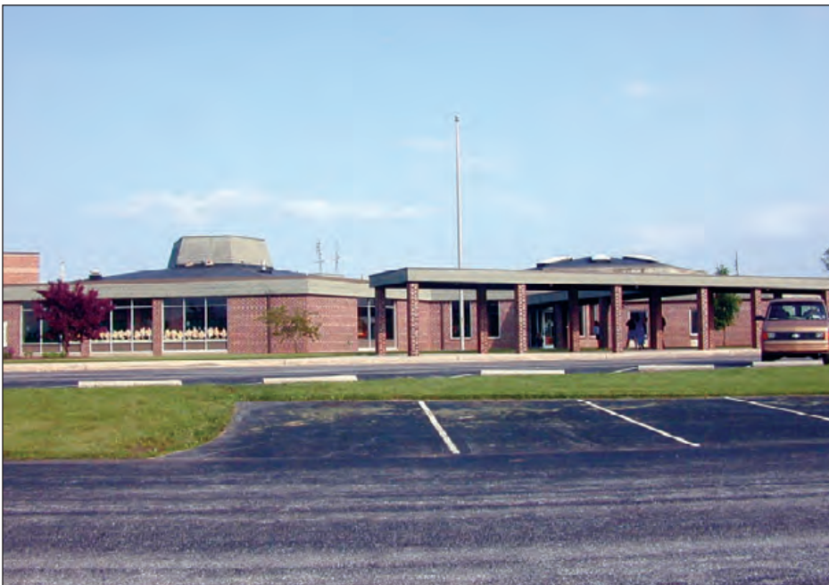
Figure 1-9: Elementary school, Fairfield, PA, 1980s
