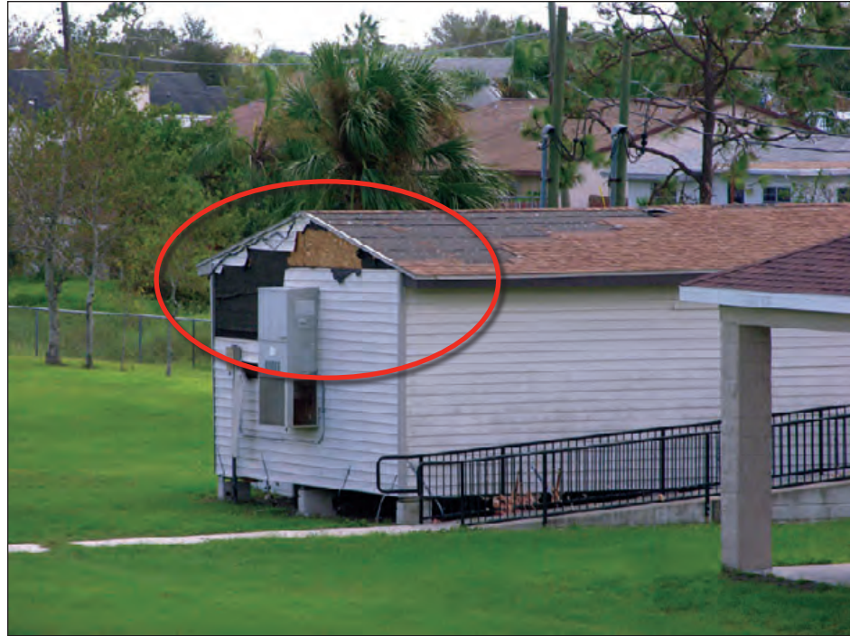
Figure 6-28: Asphalt shingles and vinyl siding blew off of this portable classroom. This type of wind-borne debris can break unprotected glazing. Hurricane Francis (Florida, 2004)
