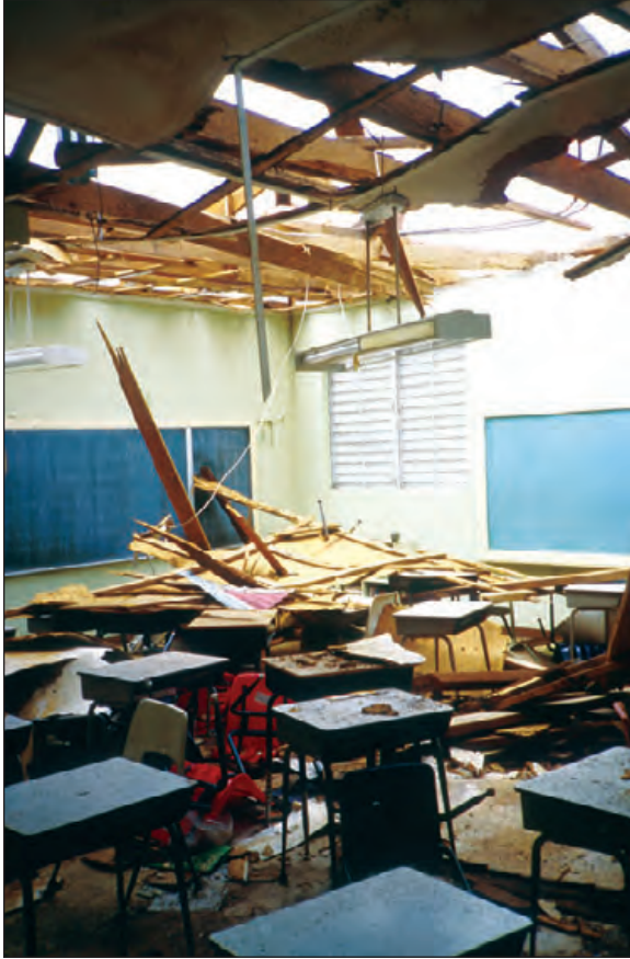
Figure 6-24: A portion of the roof structure blew off this school, and a portion of it collapsed into classrooms. Extensive water damage can cause such a school to be out of operation for a considerable period of time. Hurricane Marilyn (U.S. Virgin Islands, 1995)
