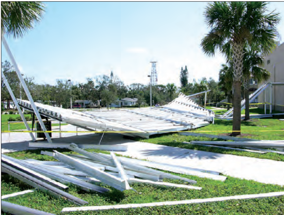
Figure 6-41: The wind speed was sufficient to collapse this school's canopy, but the speed was not high enough to blow the canopy debris very far. Hurricane Francis (Florida, 2004)
