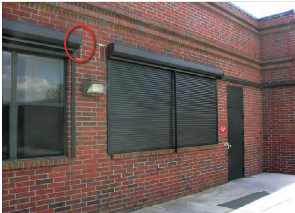
Figure 6-128: This school has roll-down shutters. The toggle in the red circle allows the shutter to be manually raised. Estimated wind speed: 130–140 mph. Hurricane Charley (Florida, 2004)
