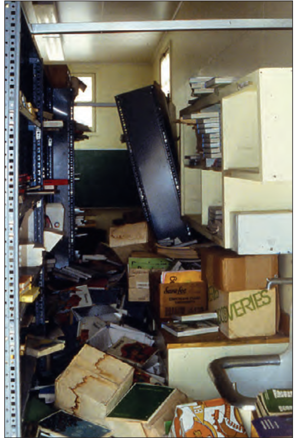
Figure 4-8: Fallen filing cabinets and shelves, Northridge, CA, 1994
