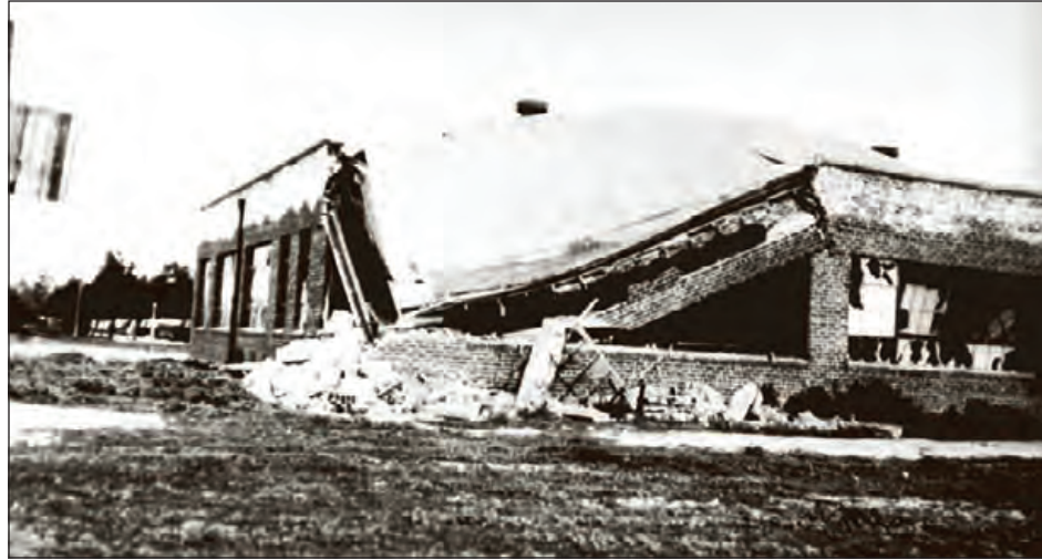
Figure 4-14: A dangerous passageway between two buildings, Polytechnic High School, Long Beach, CA, 1933
