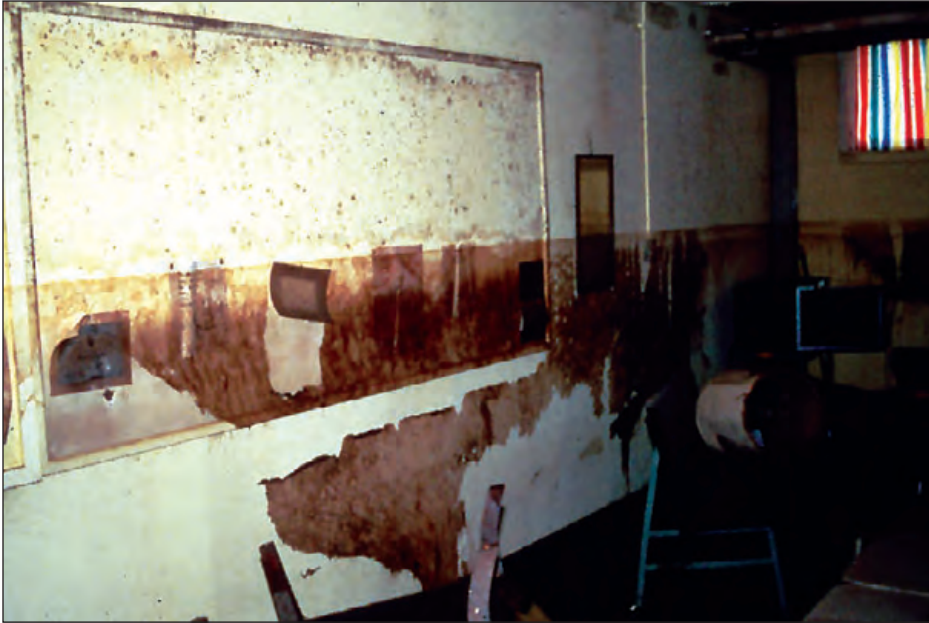
Figure 5-18: Saturation damage extends above the water line in this grade school in Gurnee, IL.
