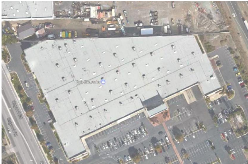
Figure C12.10.4-2. Example of a structure with non-rectangular diaphragm that is beyond the scope of the Section 12.10.4 provisions.
