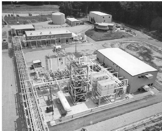
FIGURE C15.1-2 Steel pipe rack
