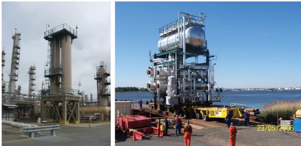
FIGURE C15.5-2 Examples of Structural Towers That are Not Integral with the Supported Tank
