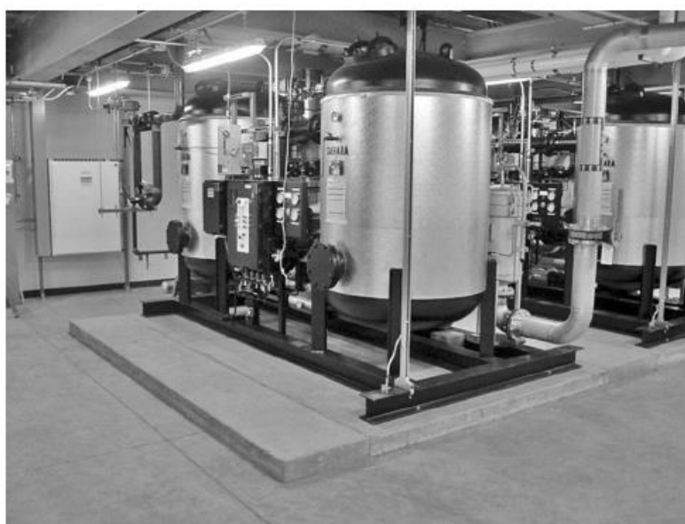
FIGURE C13.1-7 Skid-Mounted Components
