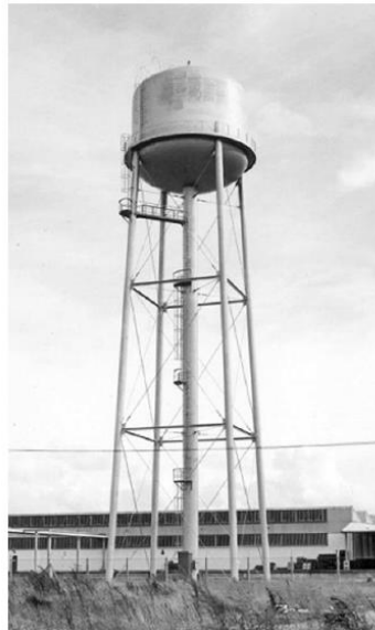
FIGURE C15.1-1 Steel multilegged water tower
