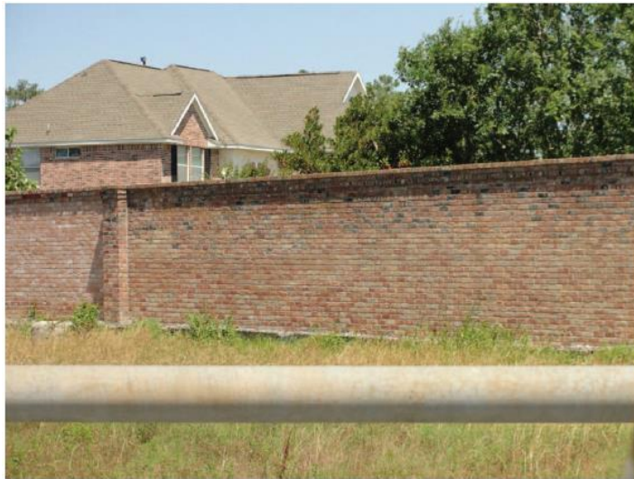
FIGURE C15.6-4 Typical Masonry Ground-Supported Cantilever Wall
