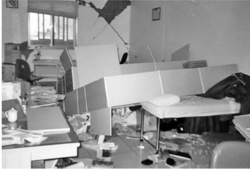
FIGURE C13.1-4 Toppled Storage Cabinets
