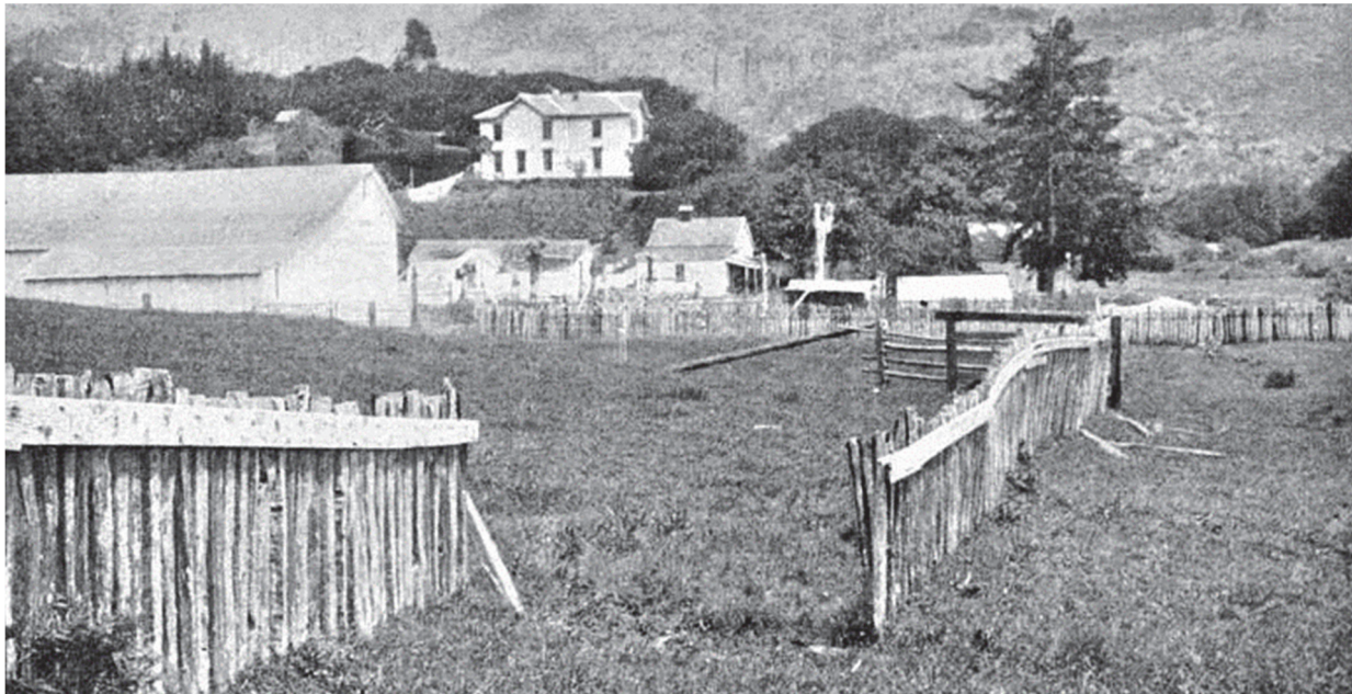
Figure 1-14 Horizontal offset of a fence near Point Reyes, California from fault rupture in the 1906 7.8M San Francisco Earthquake (from USGS).
