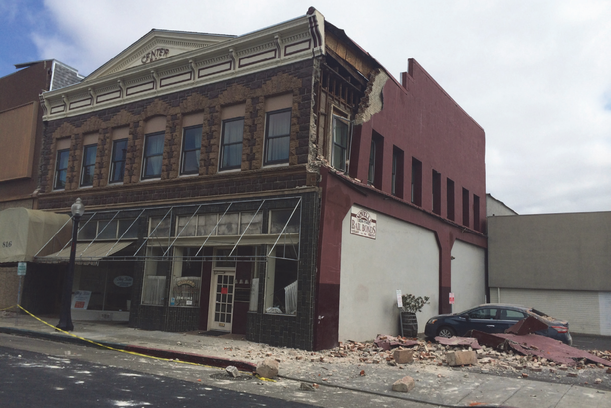
Figure 5-2 Damaged URM building in the 2014 M6.0 South Napa Earthquake (from USGS).
