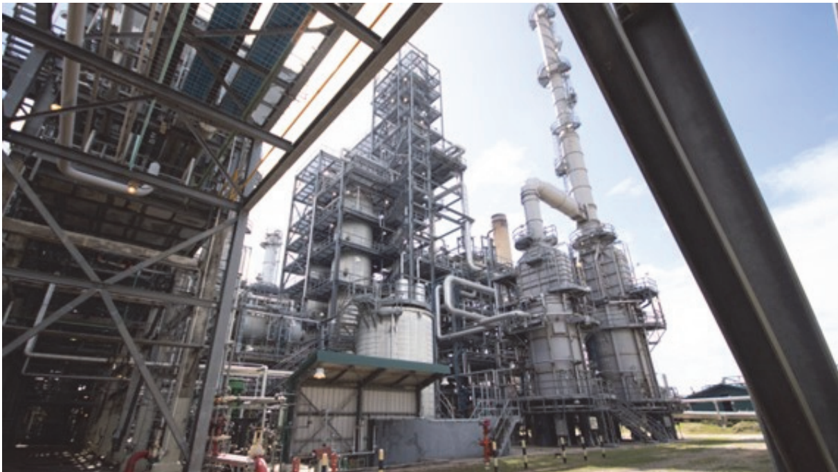
Figure 10-5 Structures commonly found in petroleum refineries and chemical plants.
