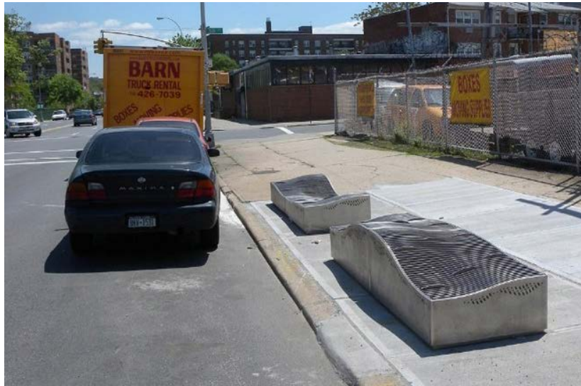
Figure 5.2.3. Elevated vent covers help protect against subway flooding while also acting as public sculptures. (Source: Jim Henderson, 2009)
