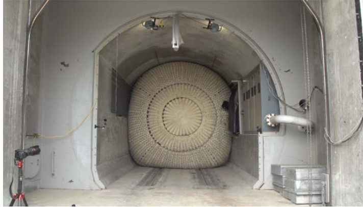
Figure 5.2.2. Inflatable plugs can prevent flooding in tunnels. (Source: Department of Homeland Security, 2017)
