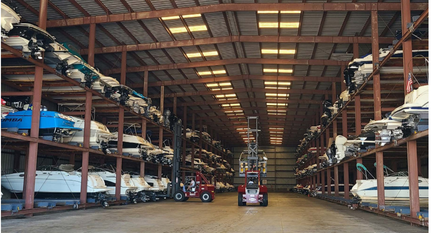
Figure 5.5.8. An example of an indoor dry-stack facility.
