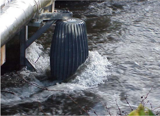
Figure 1.4.19. A debris sweeper can be attached directly to a pier to deflect debris (FHWA, 2005).
