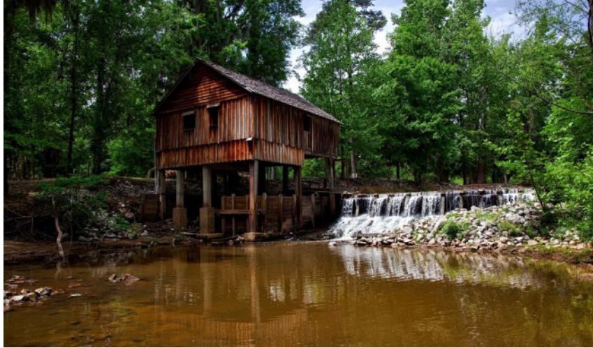
Figure 2.3.1. This dam is considered low hazard potential because, if it failed, it would only impact the forest around it. (Source: Library of Congress, Prints & Photographs Division, photograph by Carol M. Highsmith, LC-DIG-highsm-08052)
