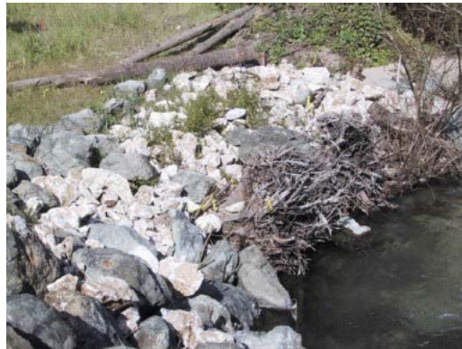
Figure 5.1.8. Nature-based solutions or hybrid approaches to streambank stabilization (combining hardscapes with nature-based solutions) can protect trails and other park facilities.
