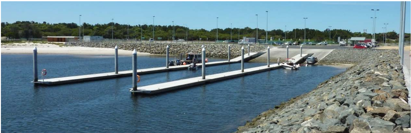
Figure 5.5.6. An example of revetments protecting a boat launch ramp system.
