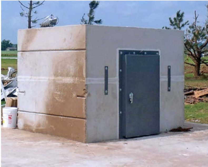
Figure 4.3.18. Data collection gateways should be protected against wind by placing them in storm shelters.
