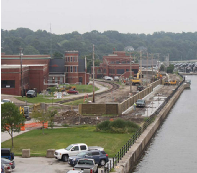
Figure 4.1.2. Constructing a floodwall around a water treatment plant can protect buildings and equipment from flood damage. (Source: U.S. Army Corps of Engineers, 2013)
