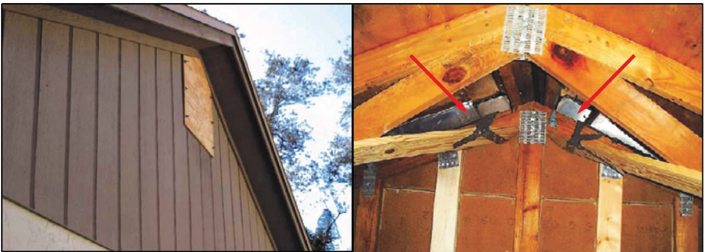
Figure 3.3.1.11. Protecting gable end vents using shutters (left) and sealing gable rake vents using metal plugs as indicated by red arrows (right).
