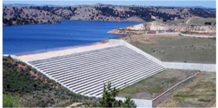
Figure 2.3.14. ACBs (left) and RCC (right) can protect spillways from overtopping erosion.
