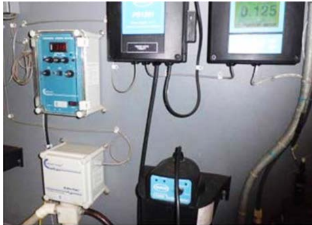
Figure 4.2.4. Elevating instrumentation can protect it from damage during flooding. (Source: U.S. EPA, 2014)
