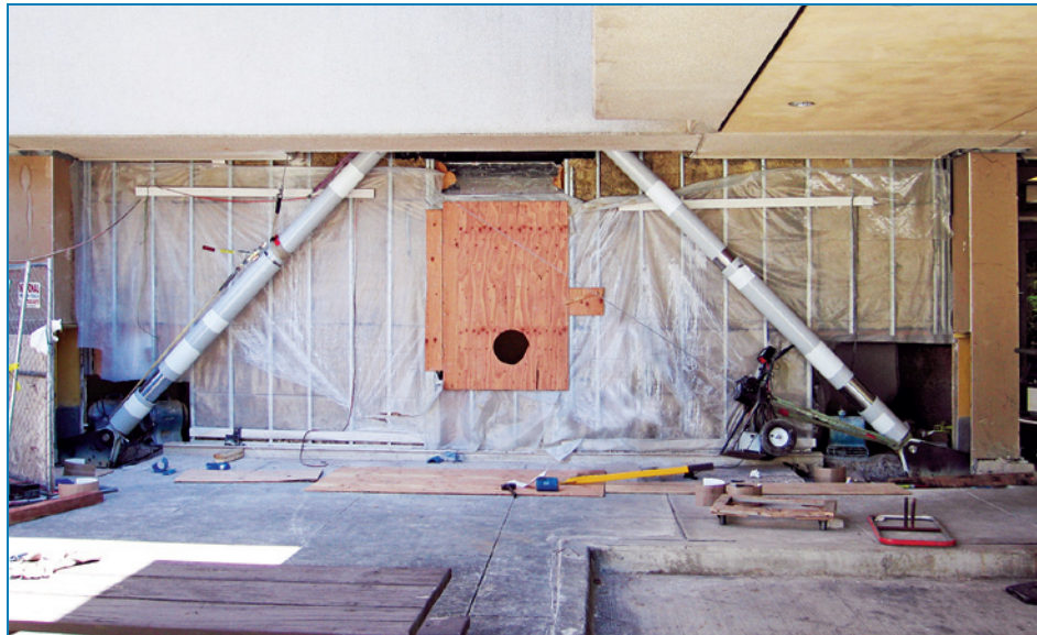
Figure 2-52: Installation of dampers at Naval Hospital Bremerton. The configuration is similar to steel braced frames.
