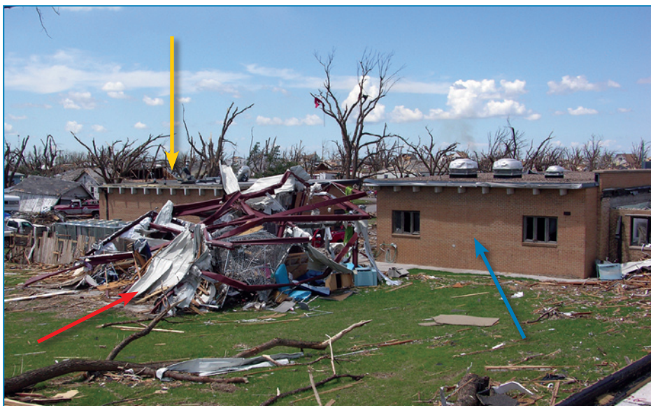
Figure 4-131: The building housing the generator is shown by the yellow arrow. The kitchen facility is shown by the blue arrow. The red arrow shows the collapsed storage building.
