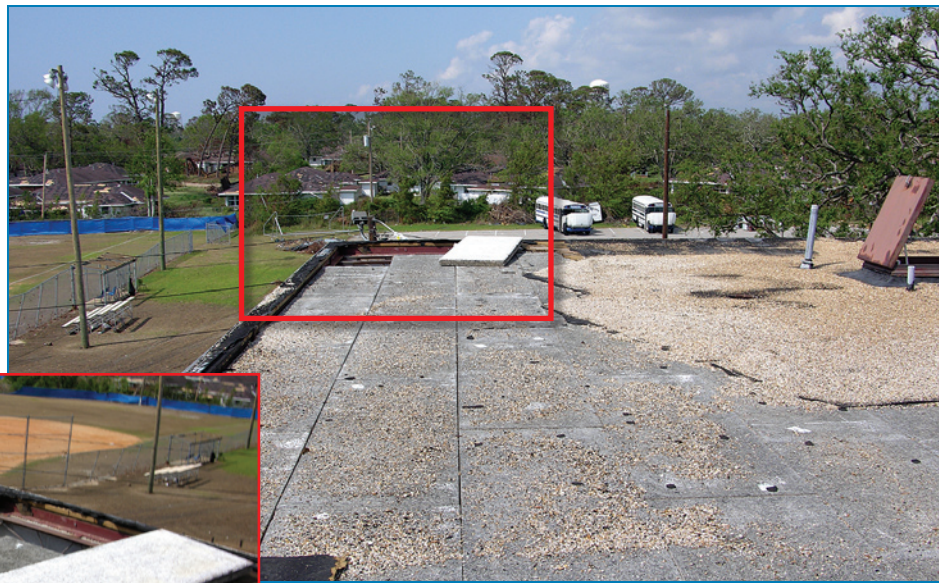
Figure 4-111: The built-up roof blew off after one of the cementitious wood-fiber deck panels detached from the joists. Hurricane Katrina (Mississippi, 2005)
