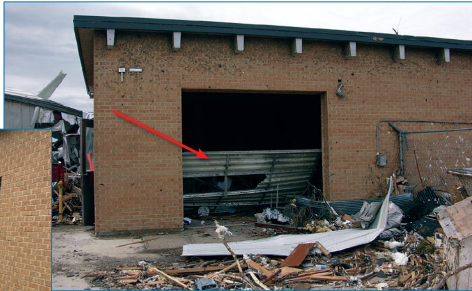
Figure 4-138: The sectional door (red arrow) at the generator building was blown in and windows were broken by debris.
