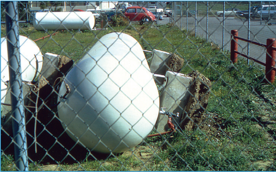
Figure 2-30: Overturned tank similar to medical gas storage
