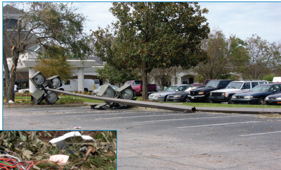
Figure 4-21: Collapsed light fixtures caused by severe corrosion (see inset). The cancer treatment facility is beyond to the left.
