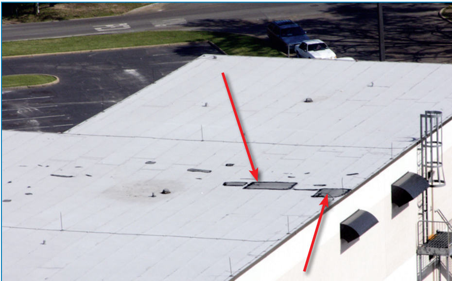
Figure 4-14: Numerous repairs where the modified bitumen roof membrane was punctured by missiles. Water from the punctured membrane entered the surgical suite.
