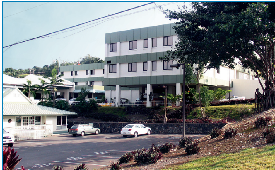
Figure 2-35: Kona Community Hospital. Addition (1989) supported on isolated columns in the foreground. The original building (1972) is in the left background.
