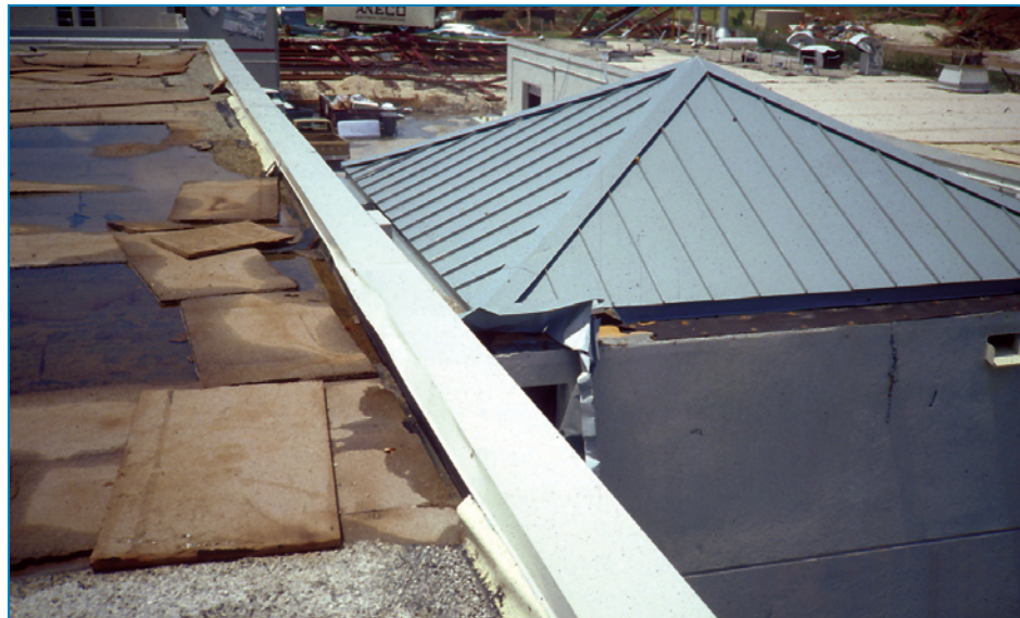
Figure 4-6: The irregularity created by the stair tower (covered with a metal roof) caused turbulence resulting in wind speed-up and roof damage. Hurricane Andrew (Florida, 1992)
