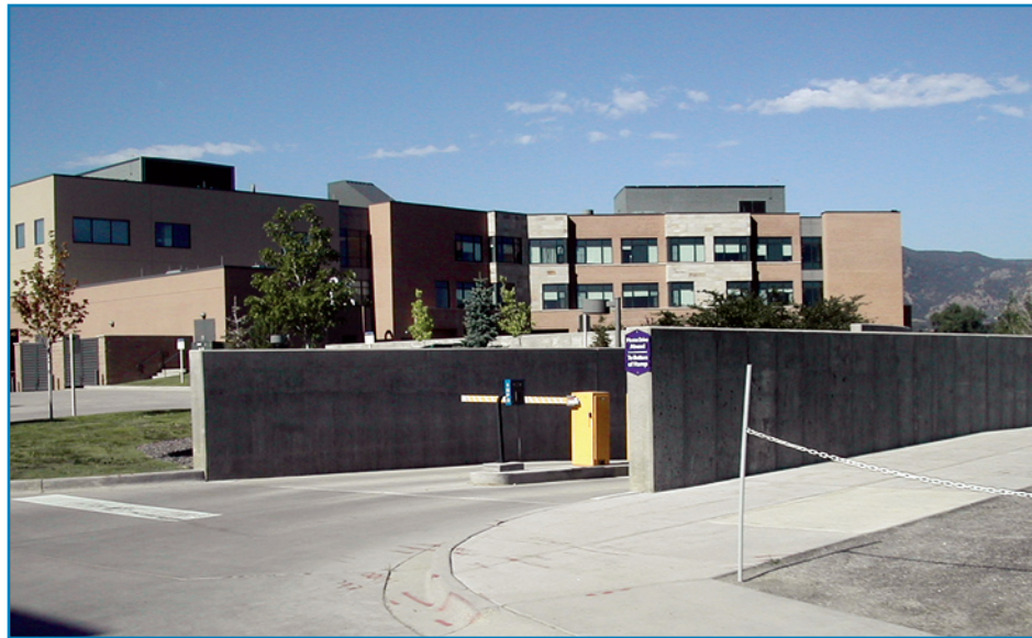
Figure 3-34: Ramp entrance to below-grade parking garage. Note retaining walls on either side; ramp crests at about 16-inches above the 500-year flood elevation.
