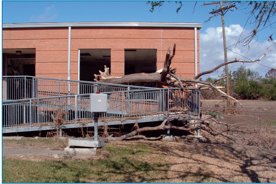
Figure 3-16: The South Cameron Memorial Hospital, Cameron, LA, was damaged by debris carried by Hurricane Rita's storm surge (2005).
