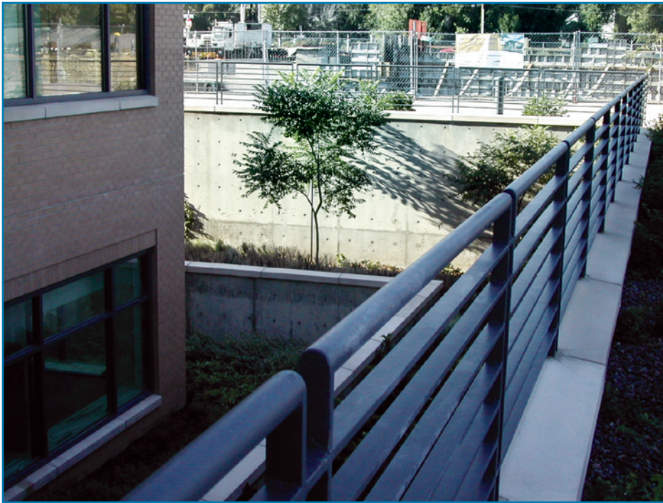
Figure 3-33: Below-grade office spaces provide natural light by construction of reinforced moat designed to provide flood protection for a foot above the 500-year flood elevation.
