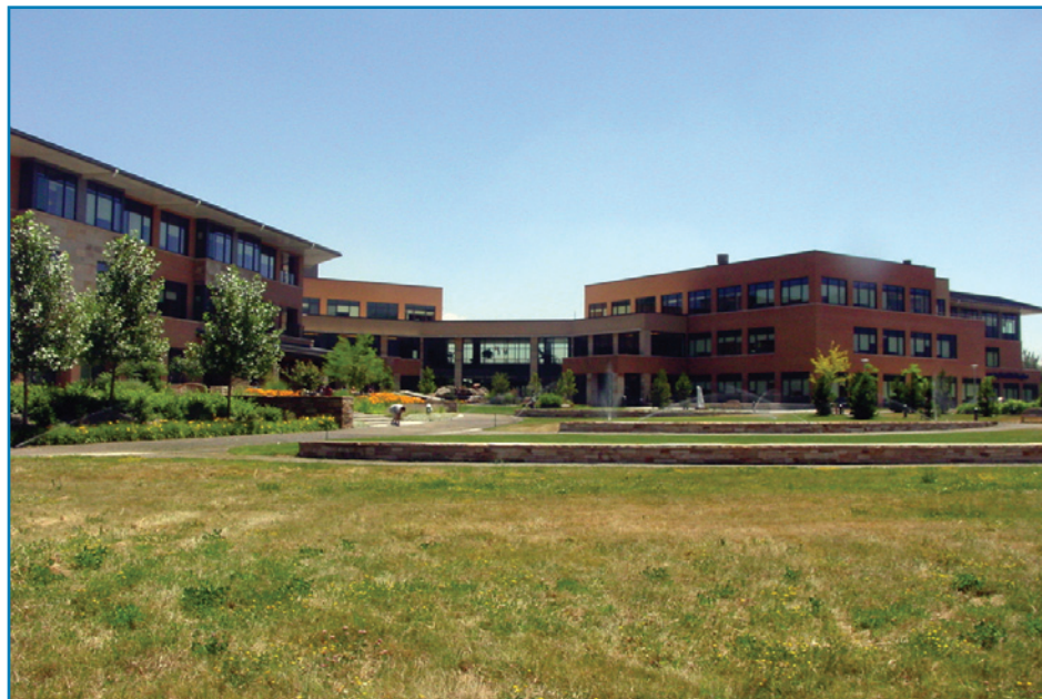
Figure 3-32: Boulder Community Foothills Hospital main entrance, with landscaping and retaining walls for portion of site filled to the 500-year flood elevation (Boulder Creek is behind photographer).
