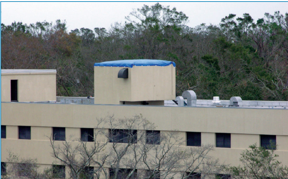
Figure 4-127: An emergency roof covering had been installed over the elevator penthouse at the psychiatric hospital.
