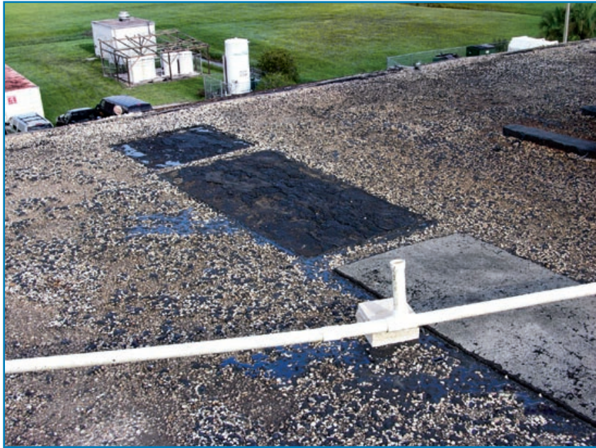
Figure 3-92: To avoid walkway pad blow off, as occurred on this hospital roof, walkway pads are not recommended. Hurricane Charley (Florida, 2004)
