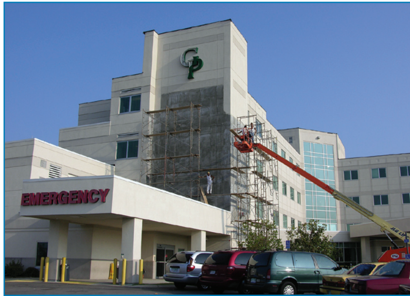
Figure 4-6: Repair of EIFS wall covering on Garden Park Medical Center
