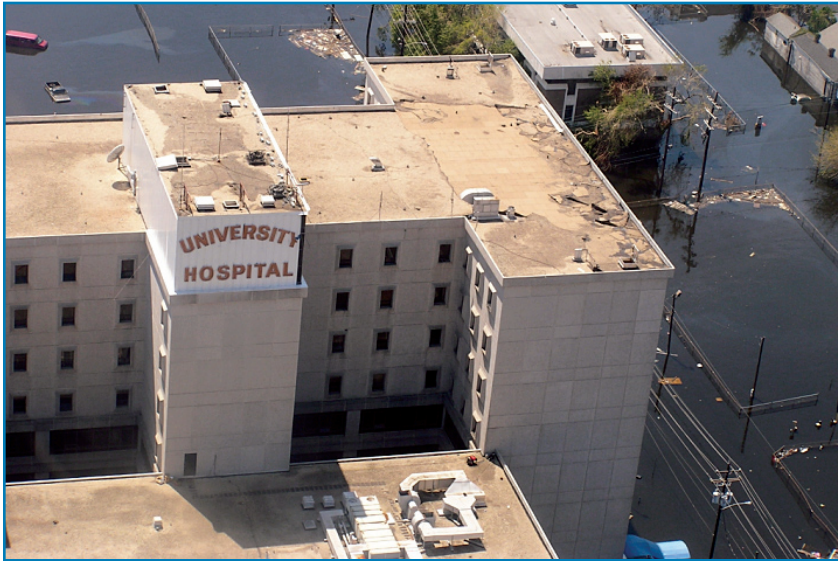
Figure 4-1: University Hospital surrounded by 4 feet of water
