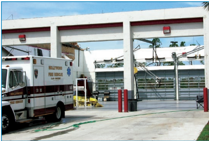
Figure 3-30: The roof structure over the apparatus bay blew off following the failure of sectional doors. Hurricane Charley (Florida, 2004)
