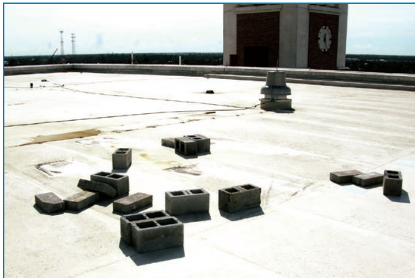
Figure 3-82: A satellite dish anchored similarly to that shown in Figure 3-81 was blown off of this five- story building. Hurricane Charley (Florida, 2004)
