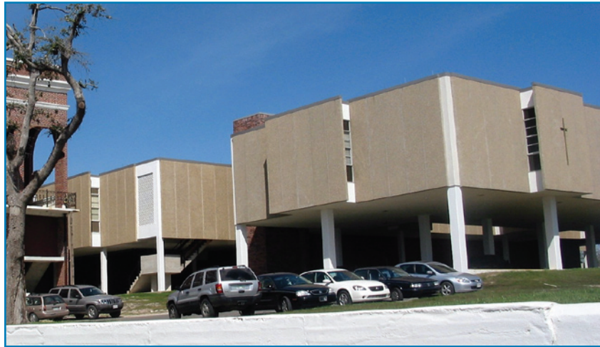
Figure 4-24: Precast concrete paneling at St. Stanislaus High School
