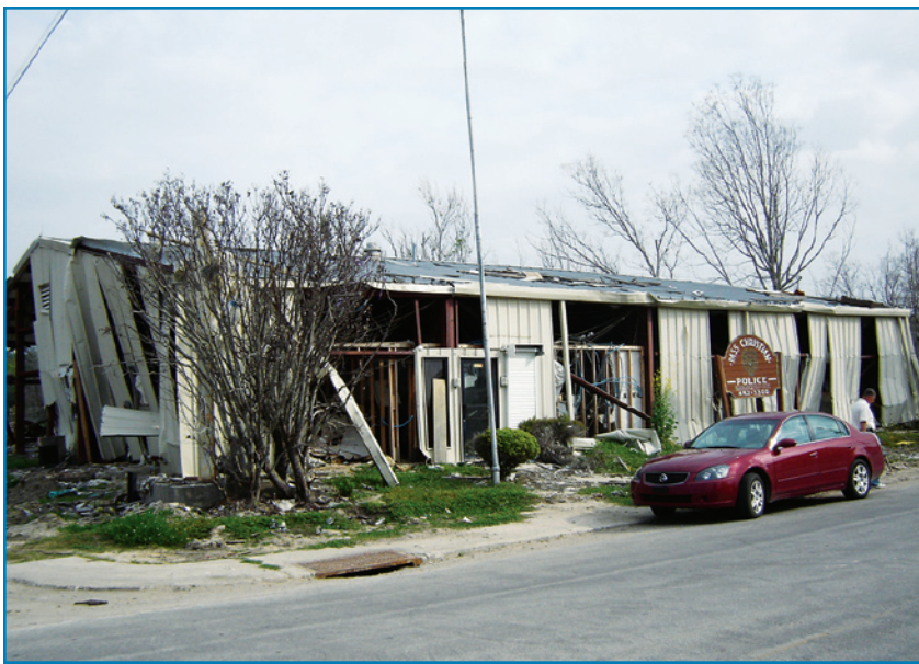
Figure 4-32: Police station in Pass Christian
