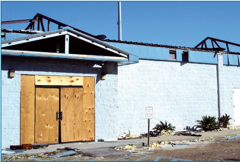
Figure 4-41: Longbeach Police Station
