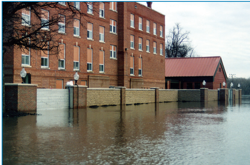
Figure 2-32: A masonry floodwall with multiple engineered openings protected the Oak Grove Lutheran School in Fargo, ND from flooding in 2001.
