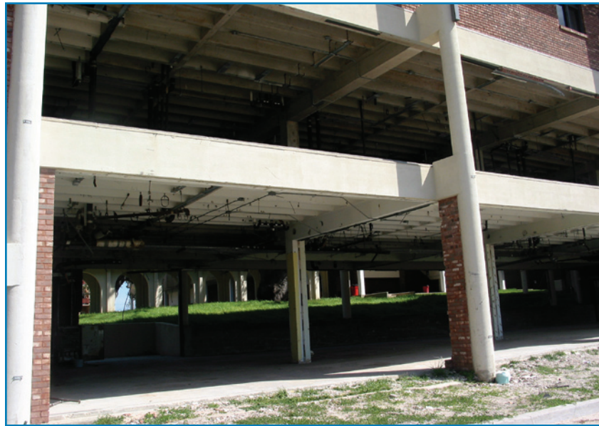
Figure 4-20: Lower floors washed away by the storm surge at St. Stanislaus campus
