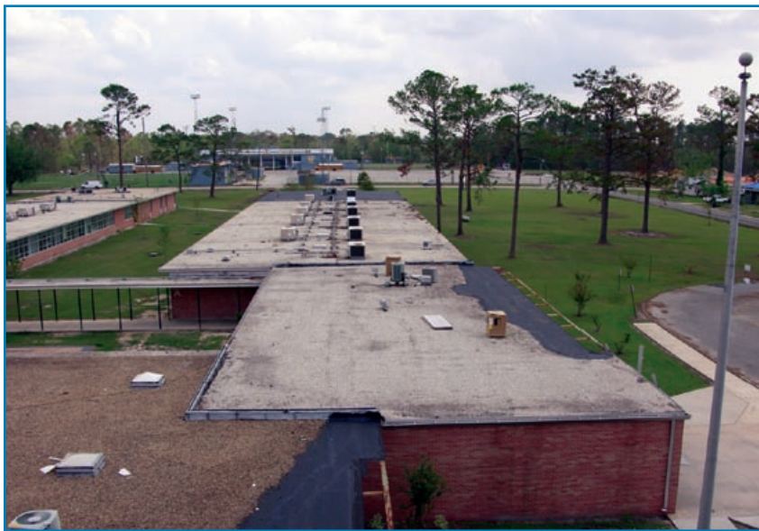
Figure 3-107: The cementitious wood- fiber deck panels detached from the joists along the overhangs and caused the school's built-up membranes to lift and peel. Hurricane Katrina (Mississippi, 2005)
