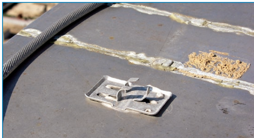
Figure 3-96: The conductor deformed the prongs under wind pressure, and pulled away from the connector. Hurricane Katrina (Mississippi, 2005)
