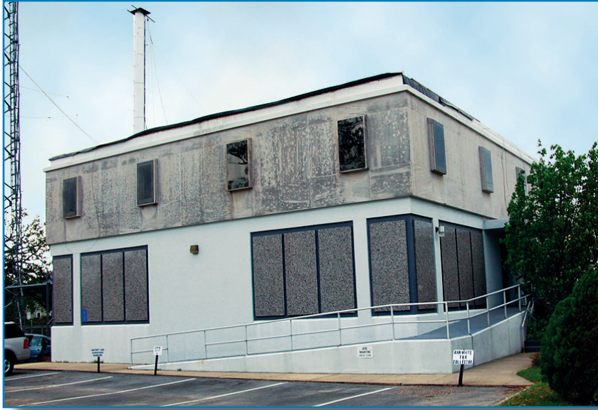
Figure 4-38: Reinforced concrete building for Jackson County EOC
