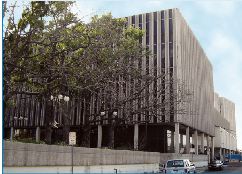
Figure 4-34: New Orleans Police Department Headquarters
