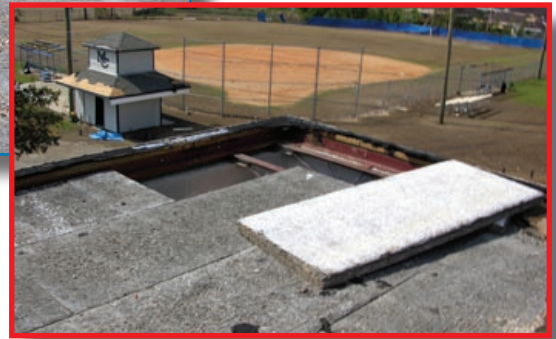
Figure 3-107: The cementitious wood- fiber deck panels detached from the joists along the overhangs and caused the school's built-up membranes to lift and peel. Hurricane Katrina (Mississippi, 2005)
