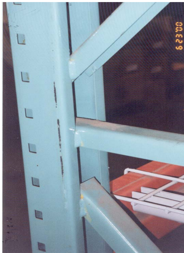
Figure 1-4 Typical rack bracing members and connections.
