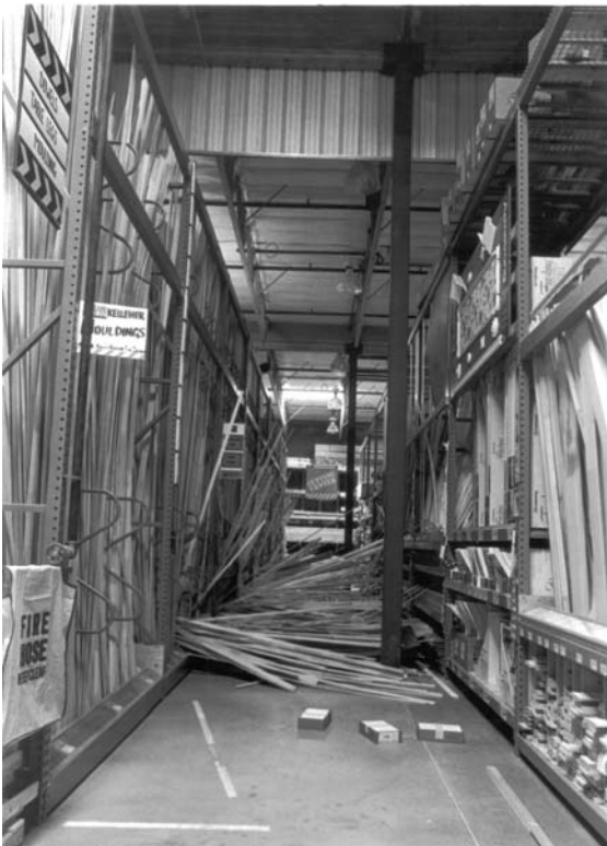
Figure 2-5 Contents spillage in the wood trim area of a Santa Clarita store.
