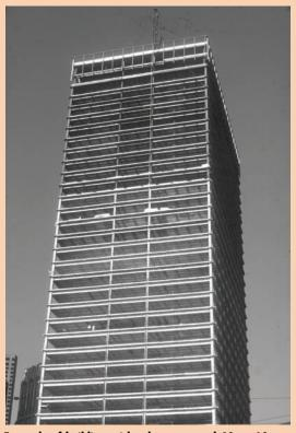
Example of building with columns spaced 40-to-60 feet apart (Option d)
