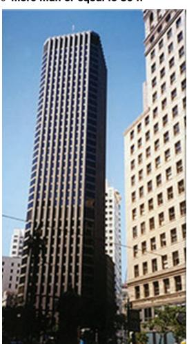
Building with columns spaced less than 15 feet apart for full height of building (Option a). Photograph courtesy of www.aviewoncities.com.
