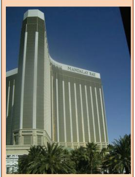
**Example three bay buildings in short direction (Option b).** A small number of bays is common for casino hotels, which typically have a single long corridor with rooms on either side on each floor.
