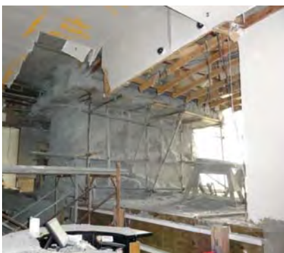
Overall View of Repair Using Shotcrete
