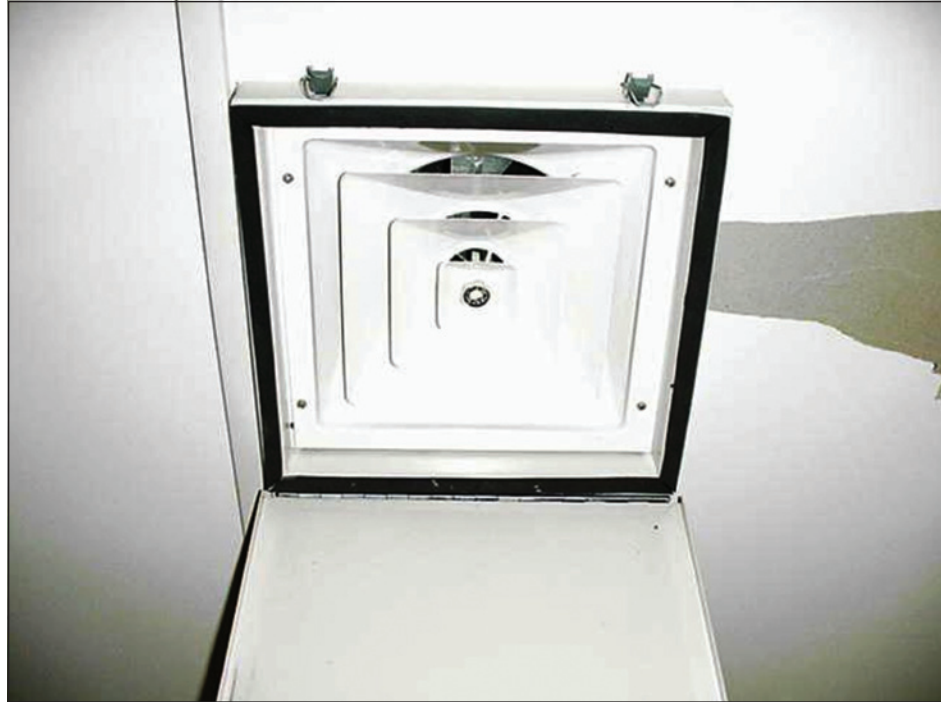
Figure 5-6: A hinged cover for sealing the supply vent of a safe room
