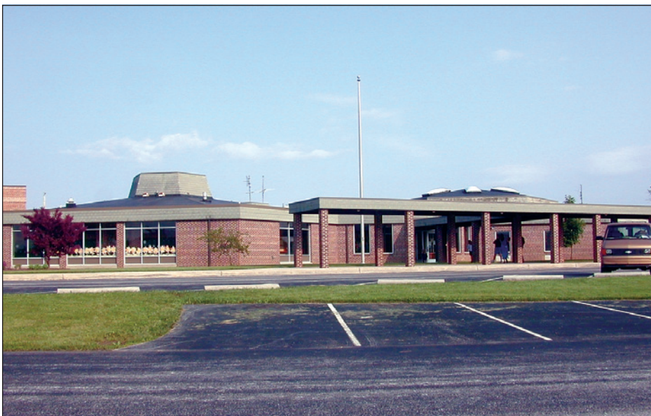
Figure 3-11: Elementary school, Fairfield, PA, 1980s
