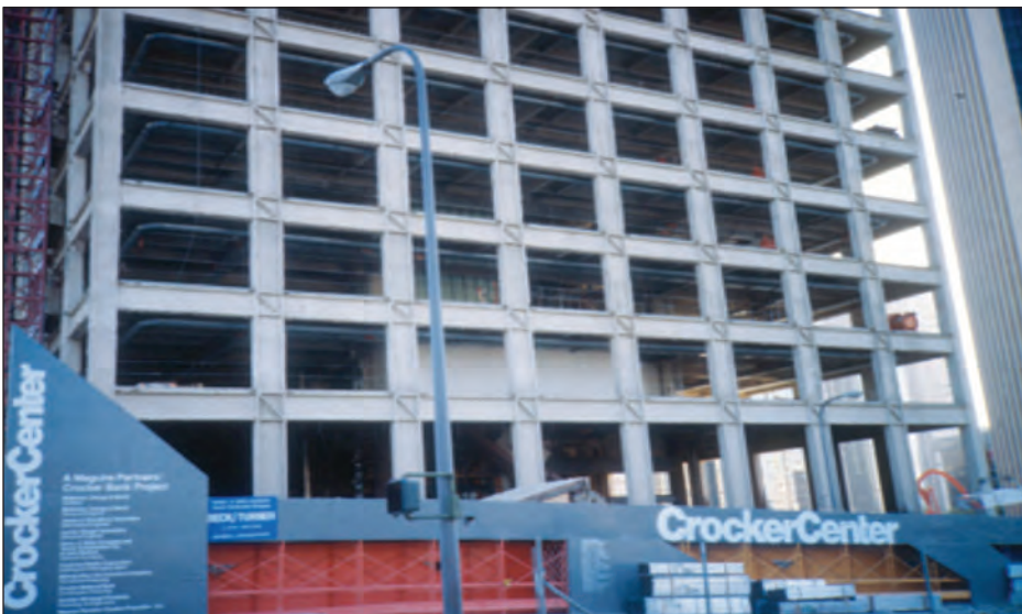
Figure 3-33: Moment-resistant steel frame structure
