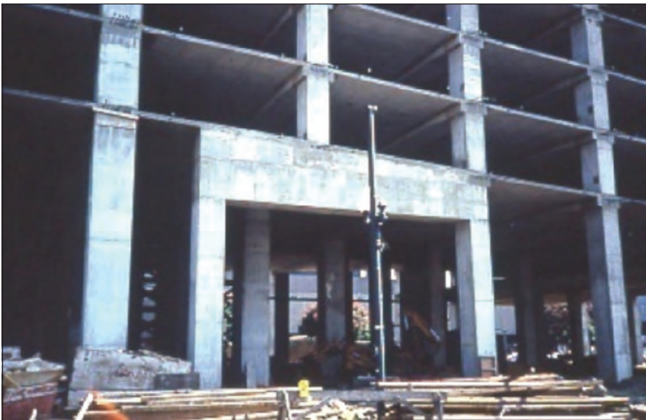
Figure 3-27: Exterior transfer girder used to provide entry at loading dock
