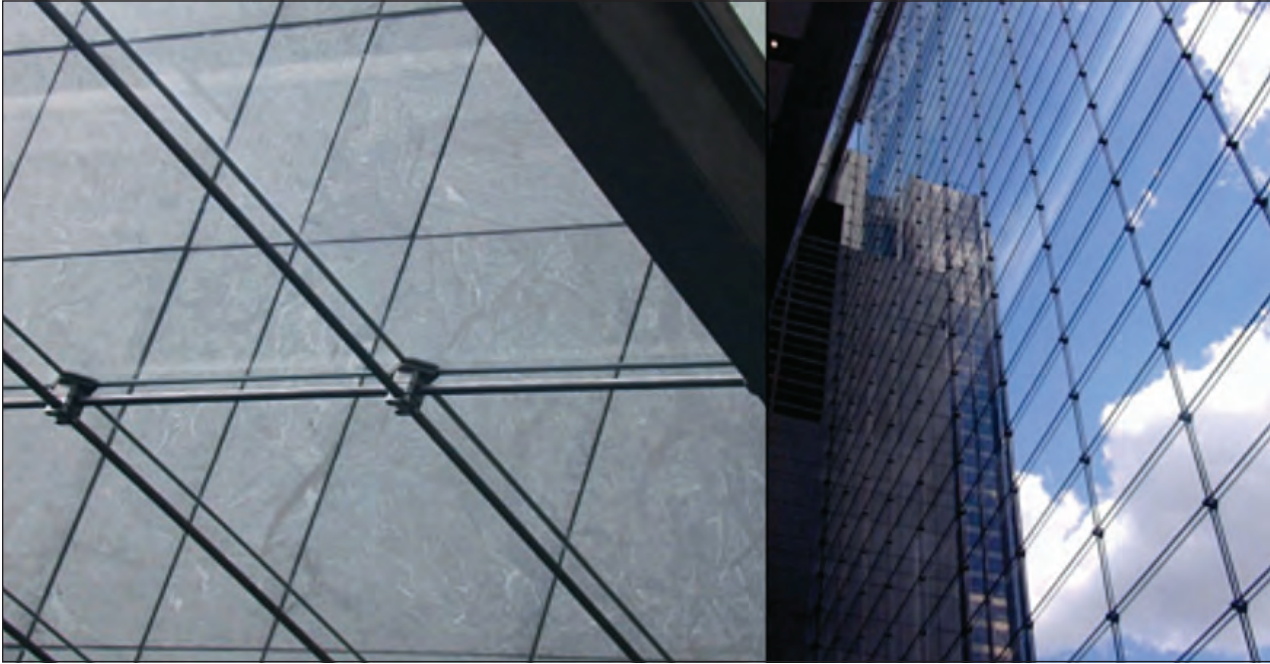
Figure 3-50: Point- and cable-supported curtain wall
