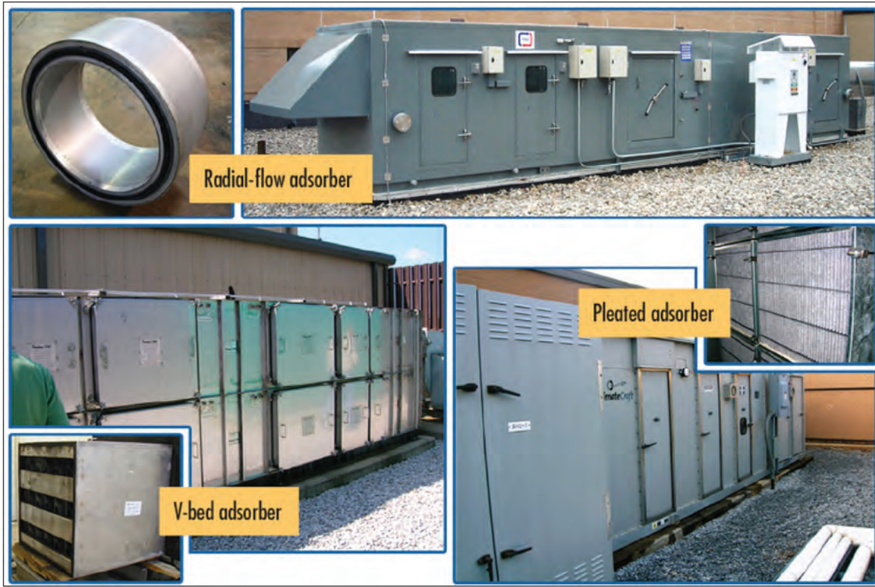
Figure 4-5: Three types of adsorbers and filter units for CBR protection of buildings
