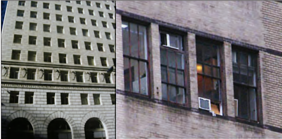
Figure 3-43: Punched windows (left), ribbon windows (right)
