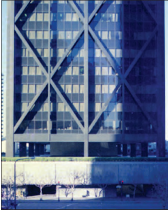
Figure 3-34: Exposed steel braced frame
