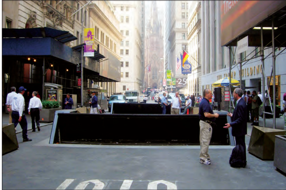
Figure 2-25: Sally port installation with two active barriers
