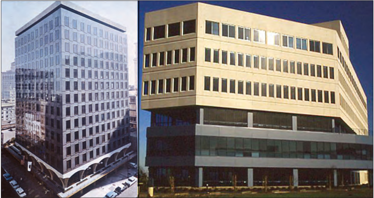
Figure 3-32: Reinforced concrete building exteriors: exterior concrete structural walls provide exterior envelope (left); reinforced concrete frame structure with nonstructural elements form the envelope (right)
