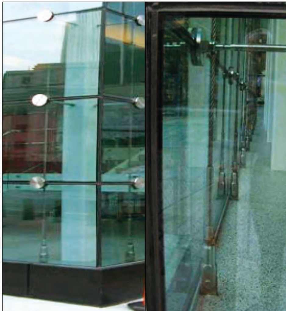
Figure 3-53: Example of cable catch system
