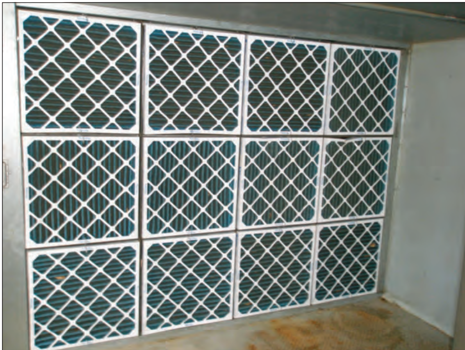
Figure 4-8: A bank of pleated MERV 8 pre-filters in front of MERV 14 cartridge filters in an office building air-handling unit
