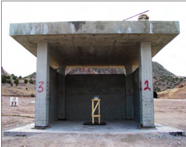
Figure 136a: Loading dock test structure.
