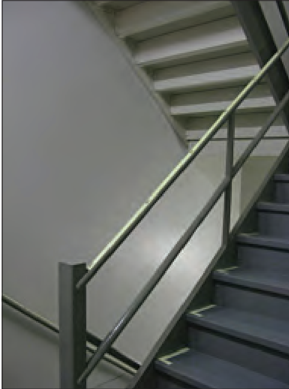
Figure 98: Example of egress stairwell
